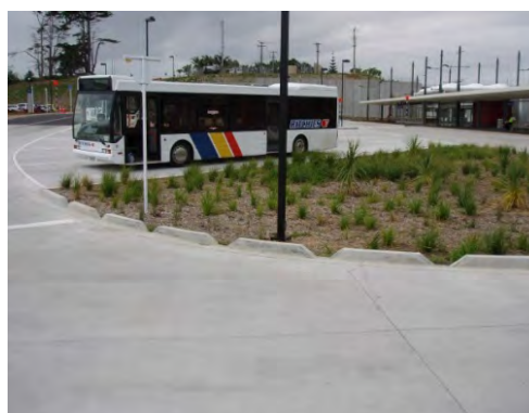
Rain garden servicing a bus depot
