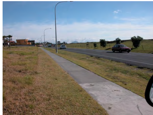
Swale in Papamoa treating highway run-off
