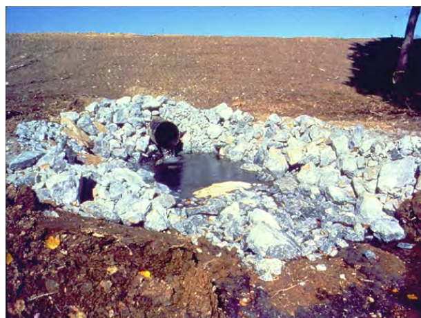
Riprap velocity dissipation at pipe outfall
