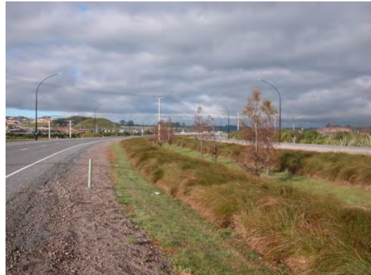
A road median with dispersed flow into vegetation (no kerb)
