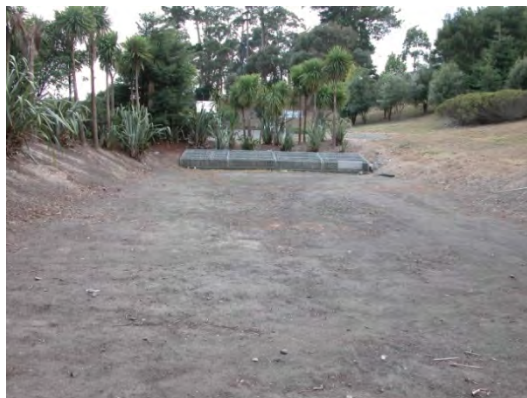
Sand filtration practice at a petrol station, recently maintained
