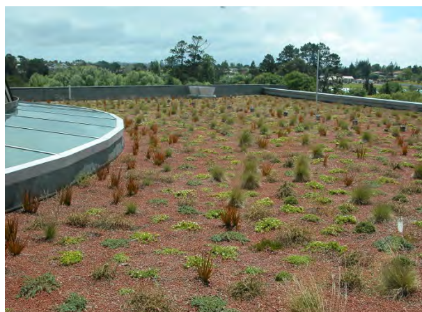
Waitakere City Council Building green roof
