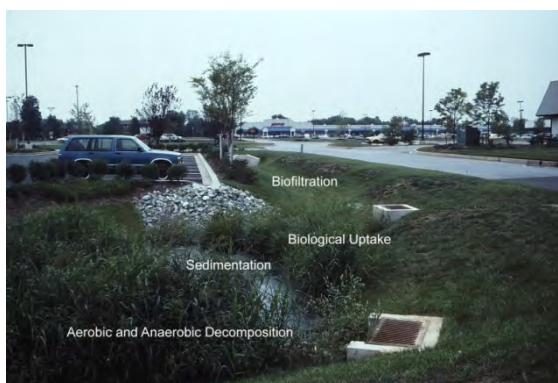
Example of treatment train of mitigation practices on one site to reduce contaminant discharge
