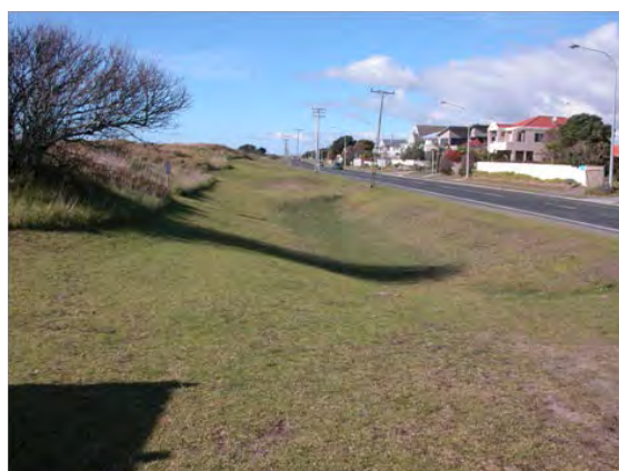
Infiltration pond in Papamoa having some pre-treatment with filter strips
