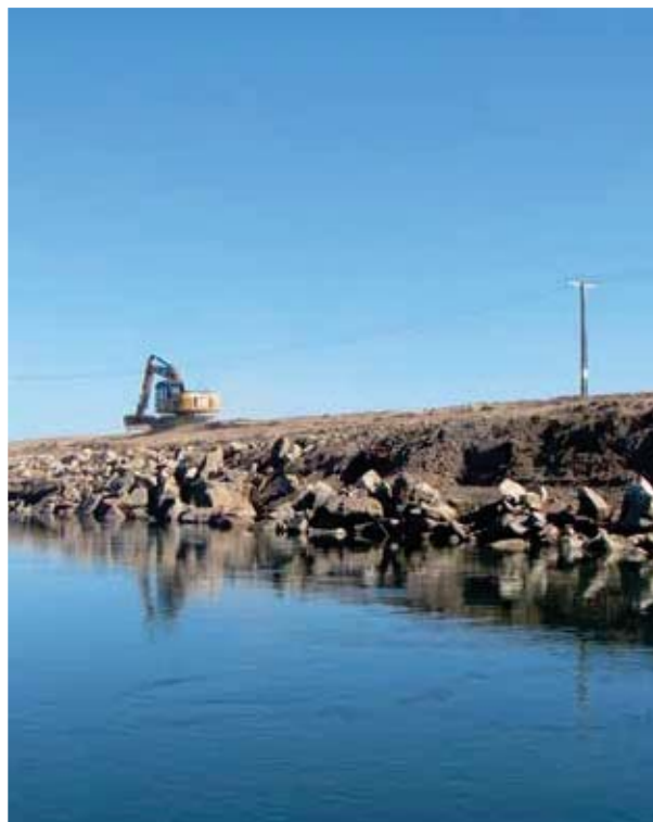
Flood works on the Rangitāiki River
