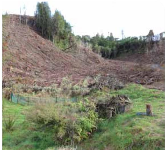
*Silt fence as final perimeter control below forestry operations.*
