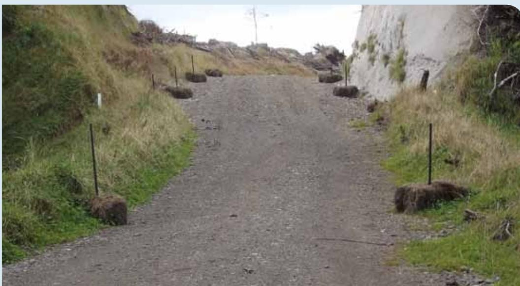
*This forestry road has a range of controls in the water tables, including metalling, grassing and using hay bales to slow down the speed of the water flow.*
