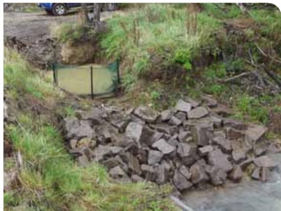
*Silt net and rock work twin culverts.*
