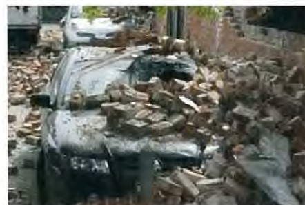
We can fall back on a disaster recovery plan to help meet costs of restoring water, sewerage and other essential services in Christchurch. Photo / Getty Images
