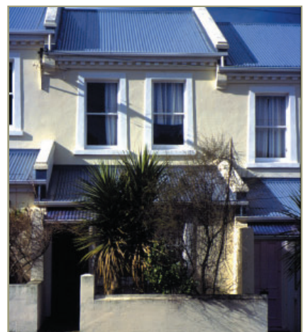
There has been a long tradition in New Zealand of housing addressing the street in a positive manner, as illustrated by these terrace houses in Dunedin.
