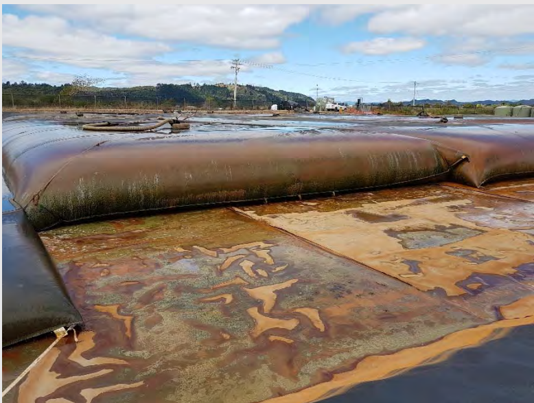
Photograph 9: Geobags within CS3 dewatering. The water coming out of the Geobags has very low turbidity and is released back into the canal.
