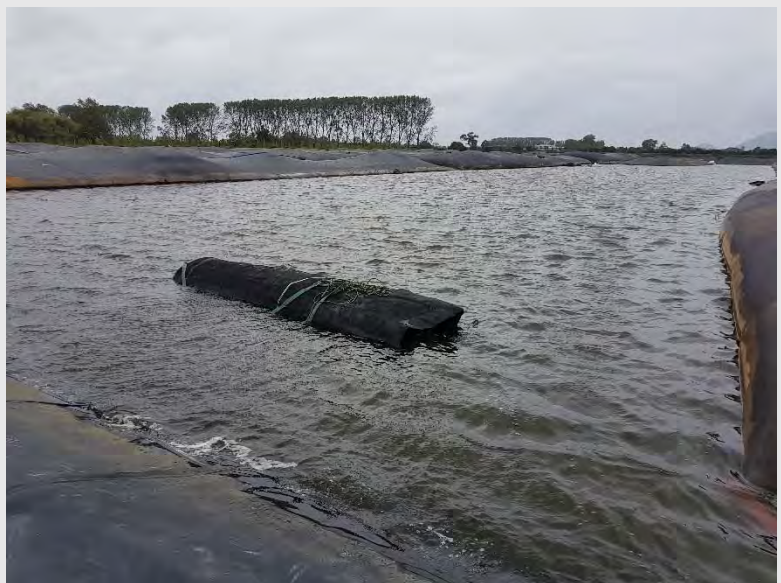
Photograph 12: CS1 flooded with rainwater.
