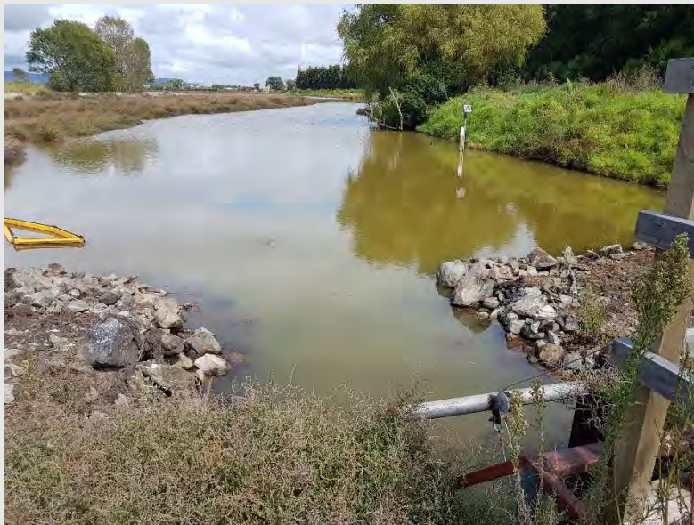
Photograph 4: FCS-East closed to maintain optimal water levels.
