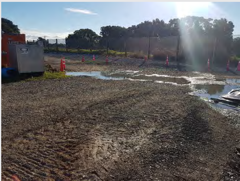
Photograph 5: A spill of potentially contaminated water outside the bunded water treatment area.
