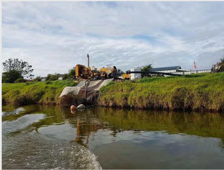
Photograph 13: Boost pump operating adjacent to Gateway Drive properties. This pump is the source of the noise complaint.
