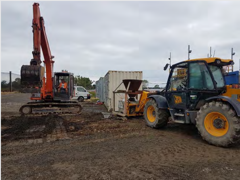
Photograph 8: Excavator scraping down the area of the spill within CS3. This material is then placed into oversized bulk bags and stored within the containment cell.
