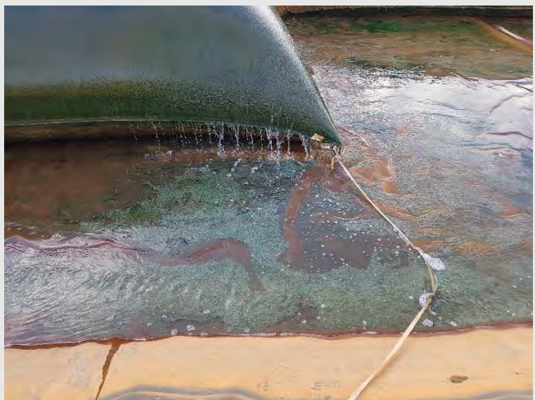
Photograph 15: Geobags dewatering at CS3. The water is clear with very low turbidity as the sediment remains trapped in the Geobags.
