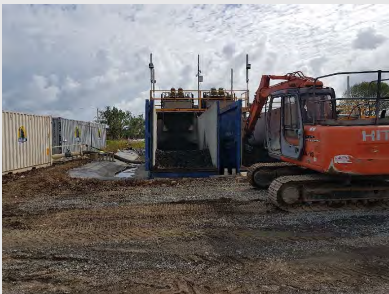
Photograph 9: Area where contaminated water spilled outside the bunded water treatment area.
