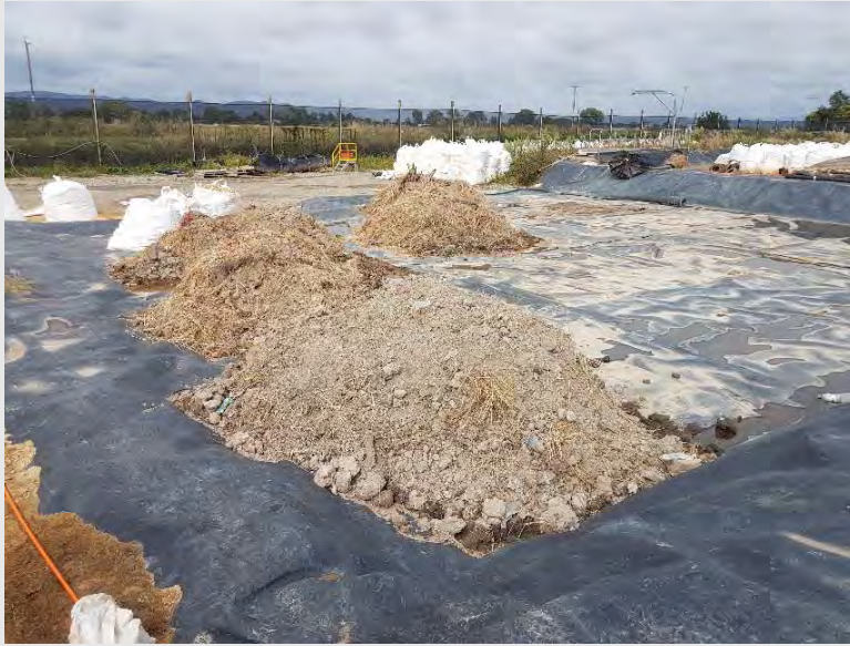
Photograph 7: Material removed from drains adjacent to Kopeopeo Canal is stockpiled within the bund at CS1. This material is not from the Kopeopeo Canal.
