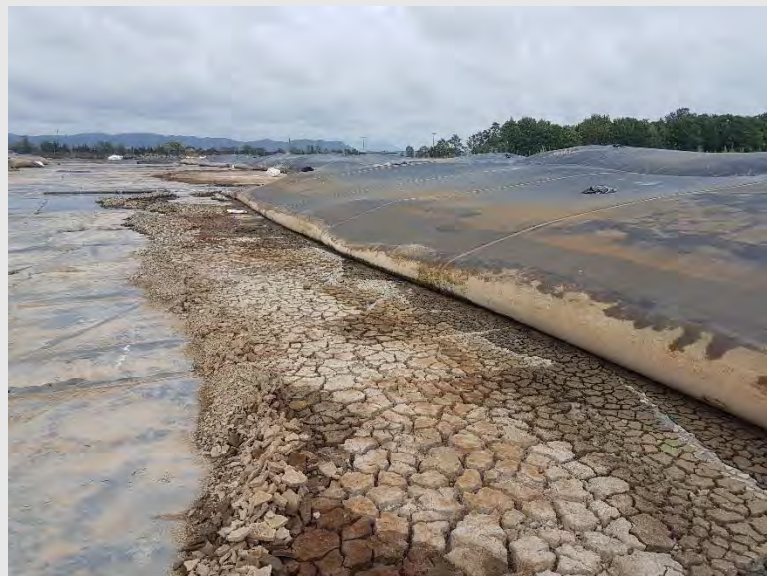
Photograph 11: Sediment dried hard within CS1 awaiting clean up.
