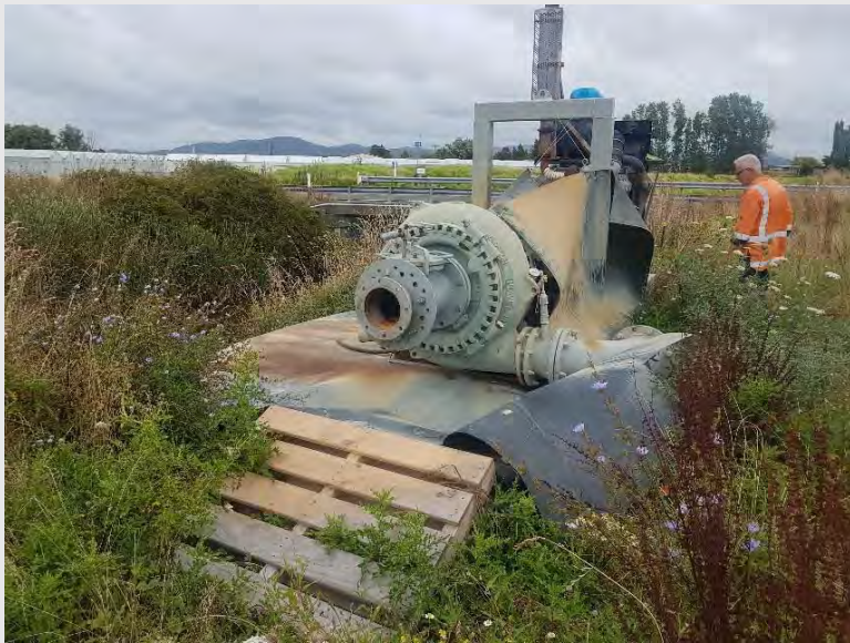
Photograph 8: Inspecting the inactive boost pump at Paroa Road.
