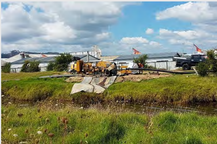
Photograph 5: Boost pump situated behind the industrial properties off Gateway Drive.
