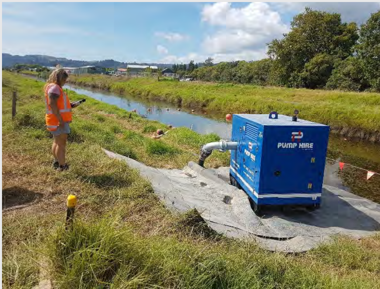
Photograph 4: Noise monitoring being undertaken at one of the boost pumps adjacent to Kope Canal Road.
