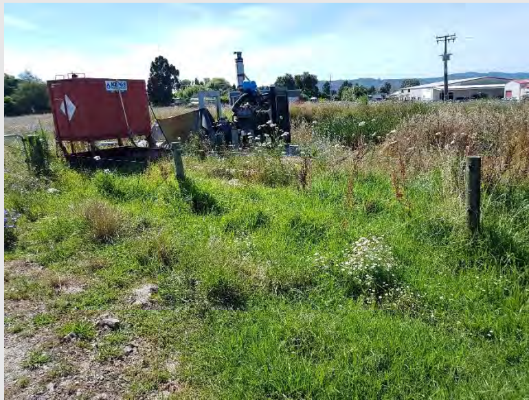
Photograph 12: Boost pump at Paroa Road awaiting removal.
