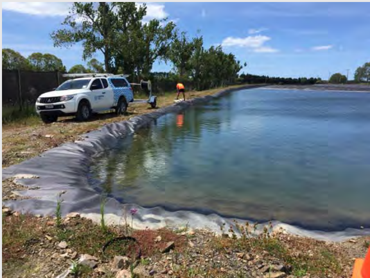
Photograph 7: Installation of monitoring and electrical equipment at CS3.
