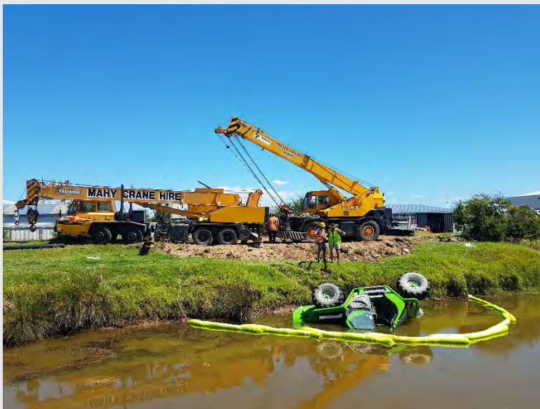
Photograph 22: Cranes setting up for lift.
