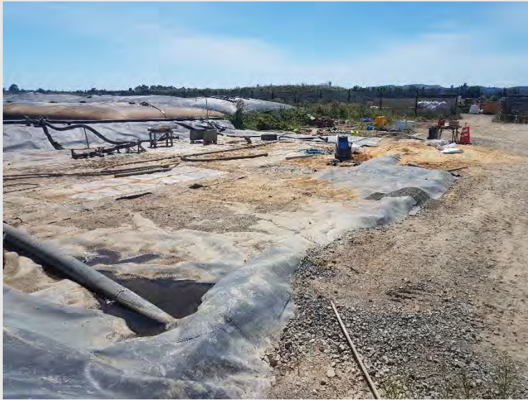
Photograph 18: CS1 water treatment area awaiting clean up.
