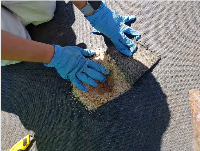
Photograph 15: Bioremediation team showing the thickness (5 to 15 cm) of the wood pellet layer on the top of the Geobags.
