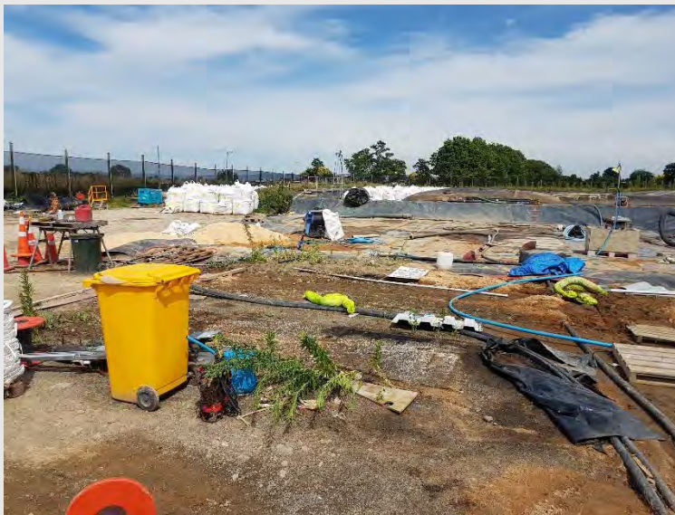
Photograph 8: CS1 during equipment move.
