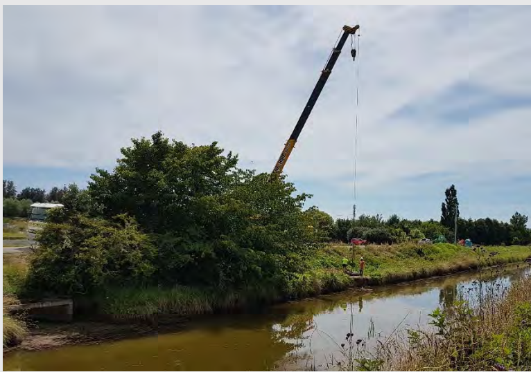
Photograph 10: Crane removing the Shaw Road boost pump.
