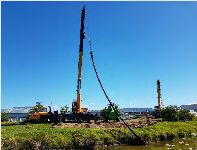
Photograph 25: Crane lifting a section of the sediment transfer pipe out of the canal.
