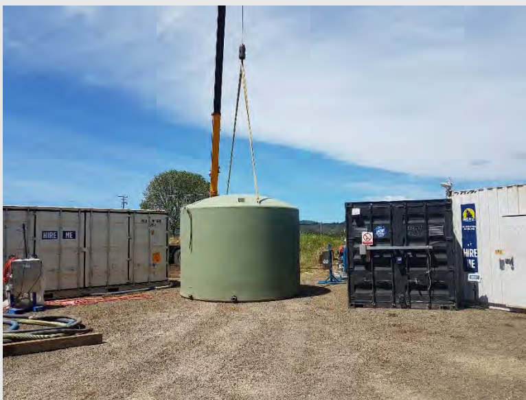
Photograph 11: Crane moving tanks at CS3.
