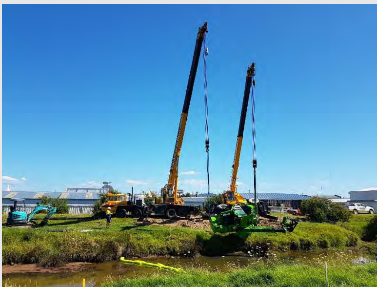
Photograph 23: Cranes lifting the Merlo out of the canal.
