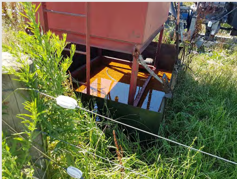
Photograph 13: Water in the bund beneath the fuel tank of the Paroa Road boost pump requiring sucker truck removal.
