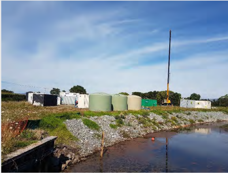
Photograph 6: Water treatment plant tanks being placed at CS3.
