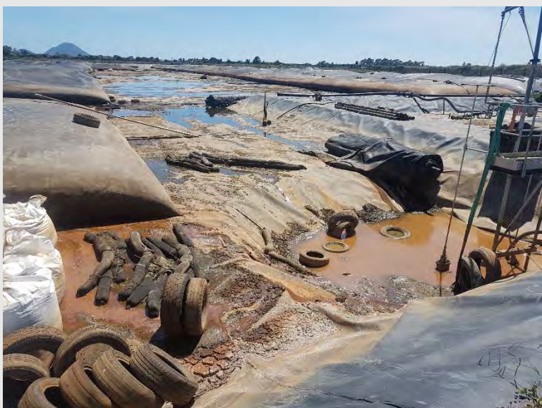
Photograph 17: CS1 sump awaiting clean up. Note the dry sediment within the containment cell as water levels are very low.
