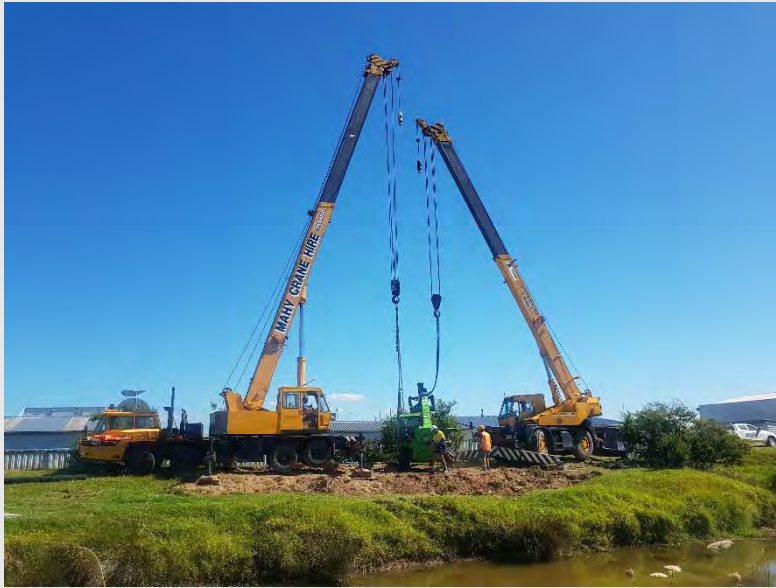
Photograph 24: Merlo having been placed on the canal bank.
