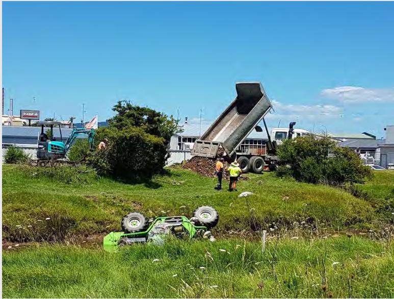
Photograph 21: Building of a temporary stable pad for the cranes to sit on while lifting the Merlo.
