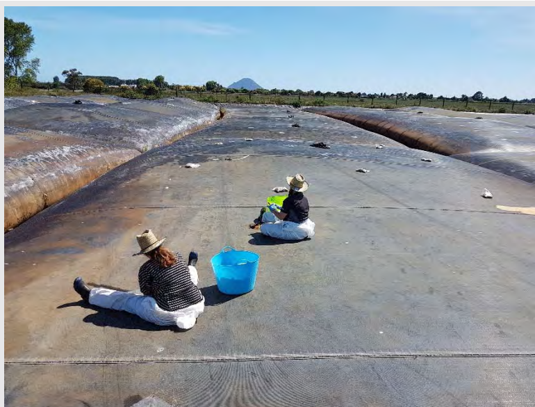
Photograph 14: Bioremediation team inoculating Geobags at CS1.
