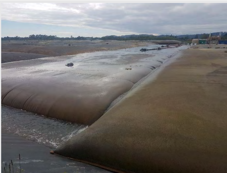
Photograph 11: A Geobag is dewatering and workers are cleaning the tops of the Geobags in the distance.
