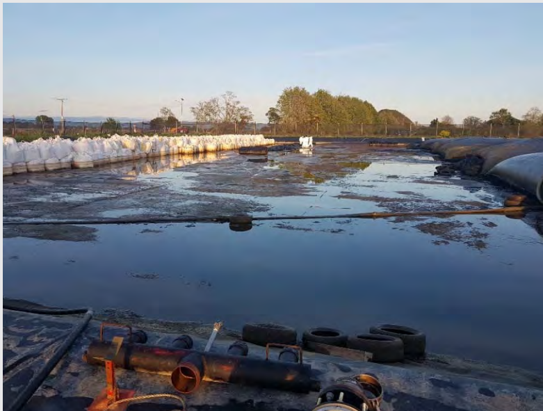
Photograph 4: Rolling out a Geobag.
