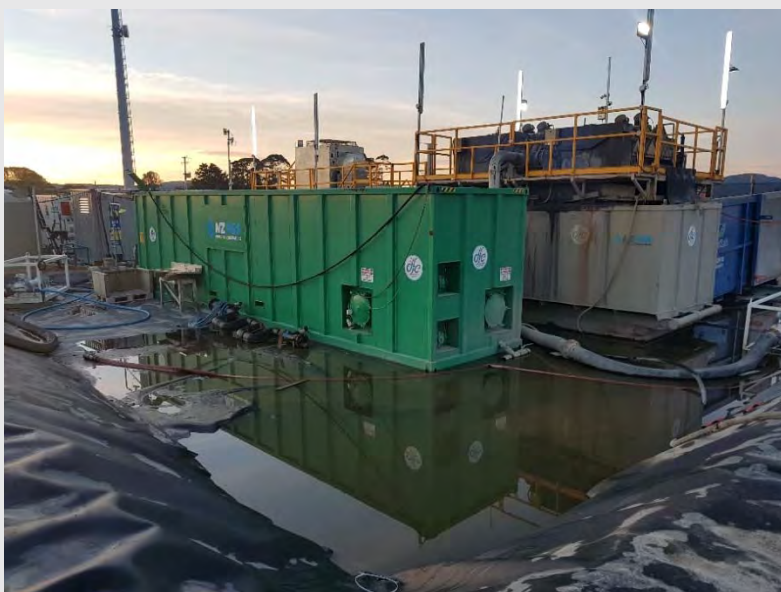
Photograph 5: Water treatment plant with water overflowing the sump but kept within the banded area.
