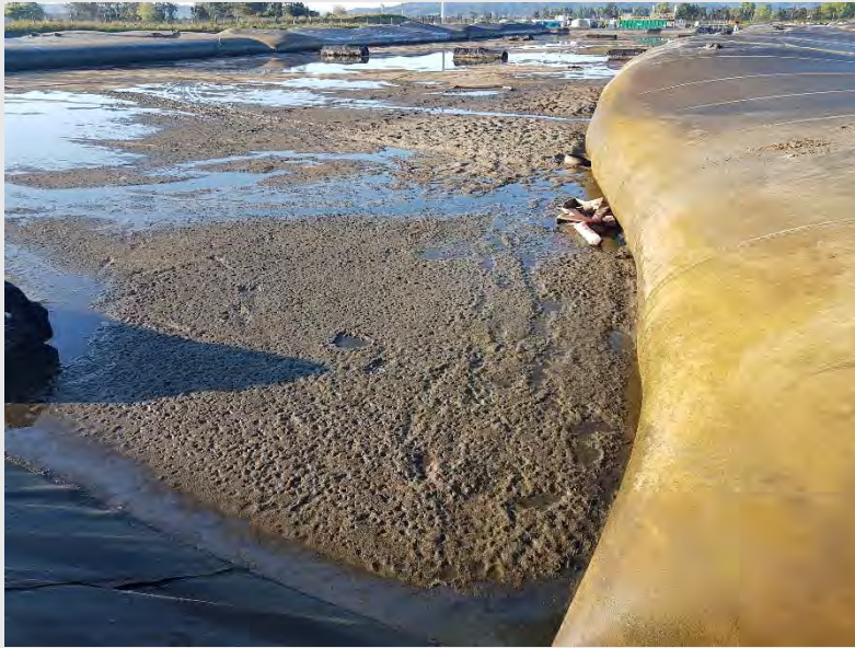
Photograph 9: Sand sitting in the containment cell is visible when the water level is dropped to allow access into the cell.
