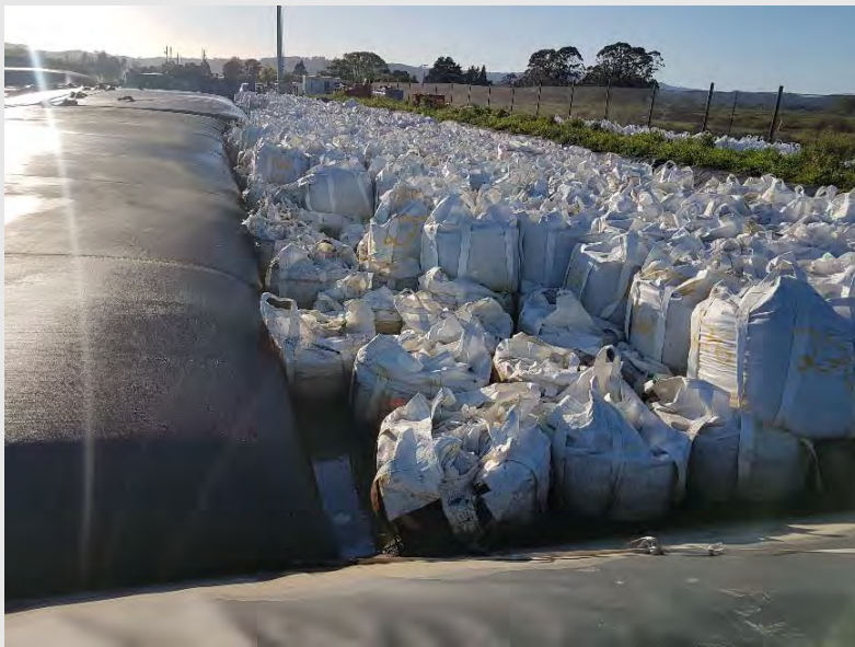
Photograph 10: Bulk bags stored within the cell. The closest one is damaged.
