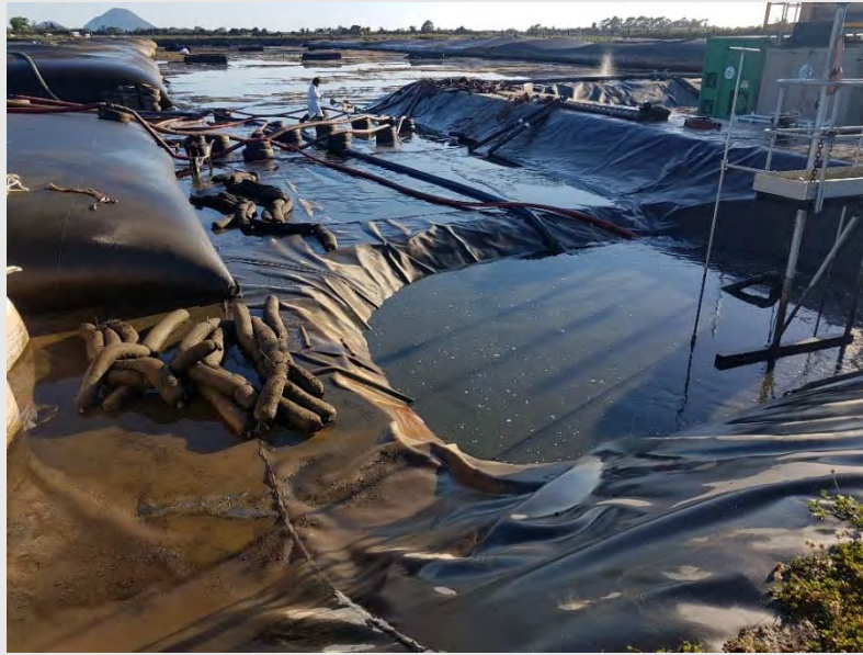
Photograph 12: The sump has had the built up sediment removed.
