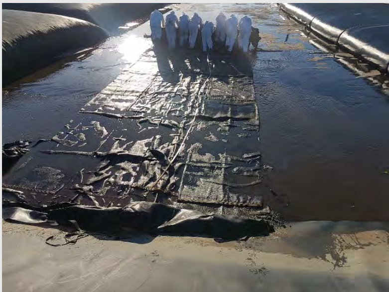
Photograph 8: Rolling out a Geobag.
