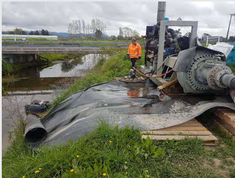
Photograph 13: Noise monitoring being undertaken around the boost pumps.
