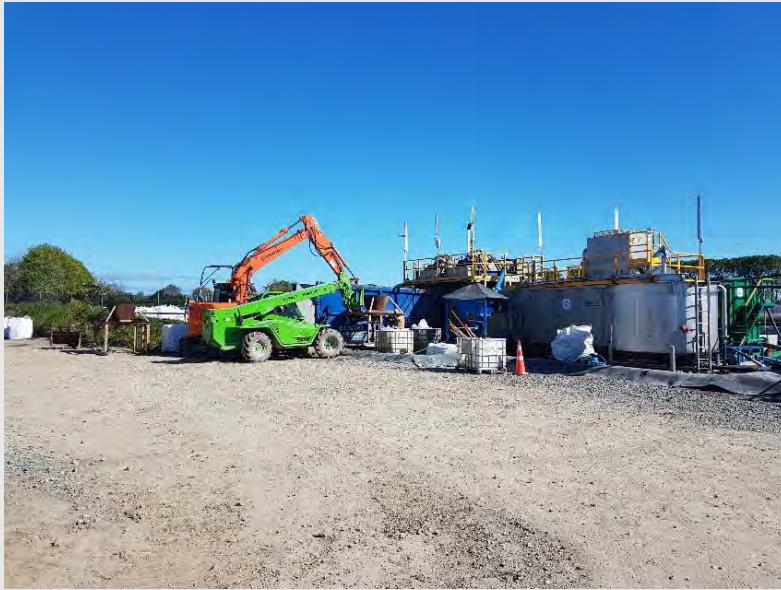
Photograph 6: Excavator moving oversized sediment from the overflow bin into bulk bags.
