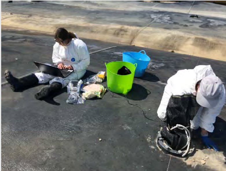
Photograph 3: Bioremediation team installing sensors within the Geobags.
