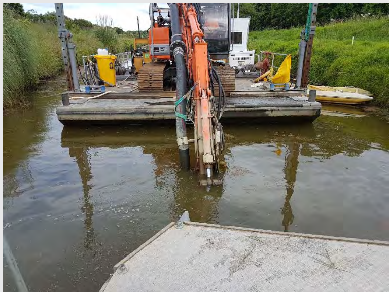
Photograph 8: Sediment sampling beside the dredge head in Section 5.
