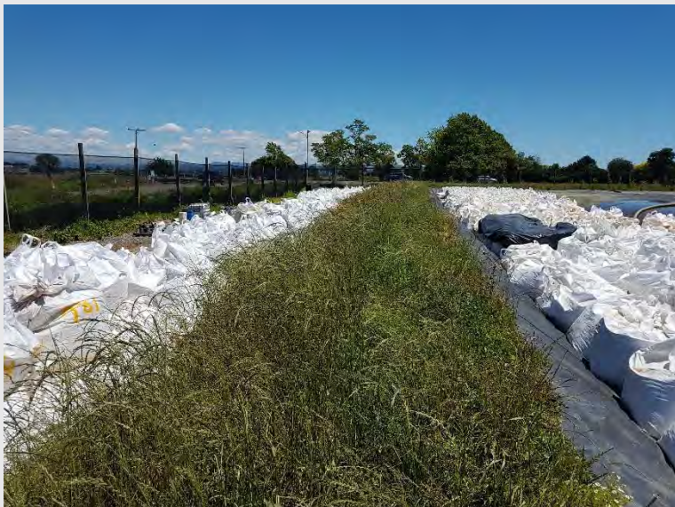
Photograph 5: Oversized material being stored before being lifted into CS1.
