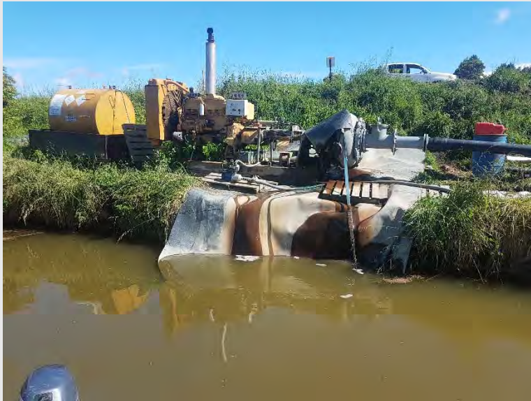
Photograph 4: Boost pump situated adjacent to Shaw Road.
