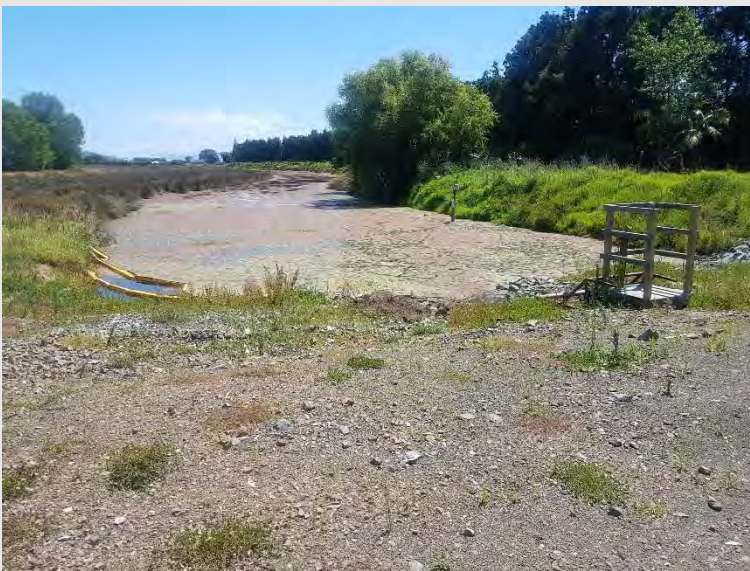
Photograph 8: Weed built up behind FCS-East.
