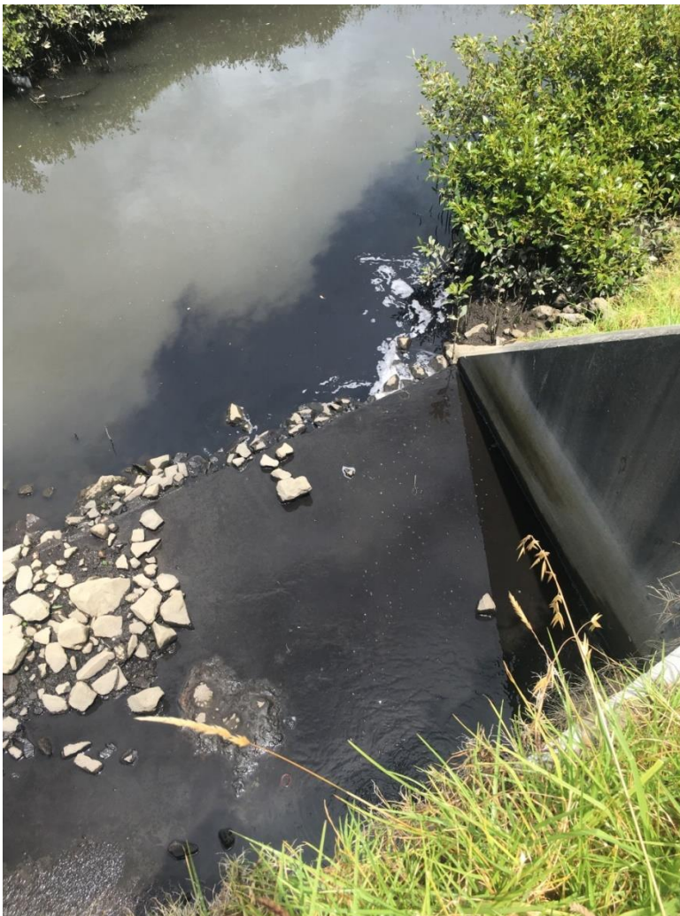
Figure 3: Point of discharge from the stormwater settlement pond into the Airport Drain.
