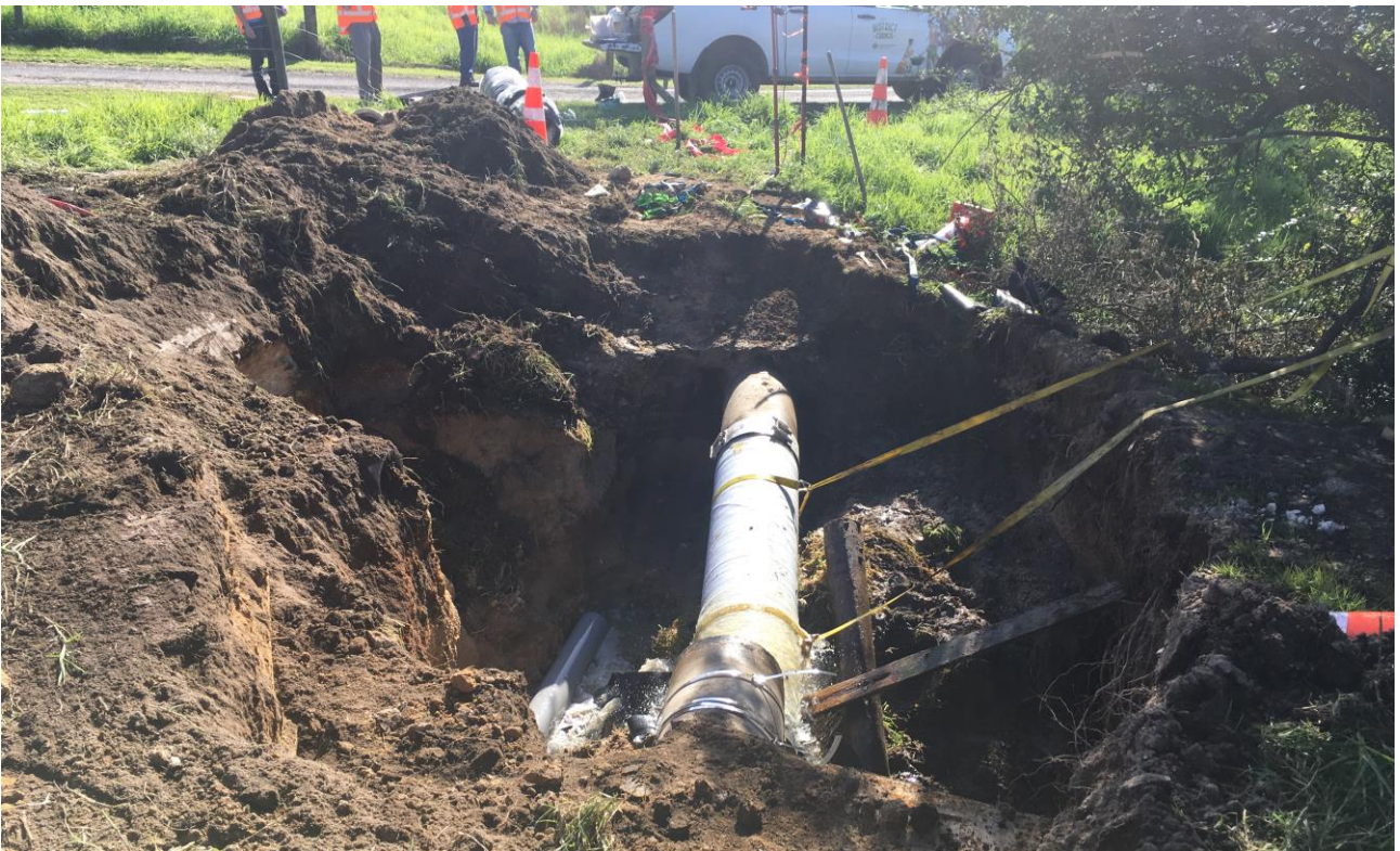
Figure 16: Pipe repair undertaken
