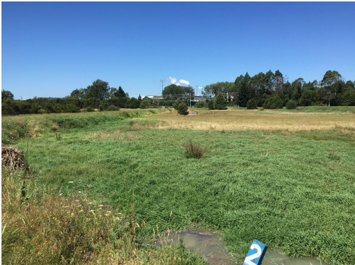
Figure 6: The RIB at Kawerau, with some pooling discharge seen to the bottom of the photo
