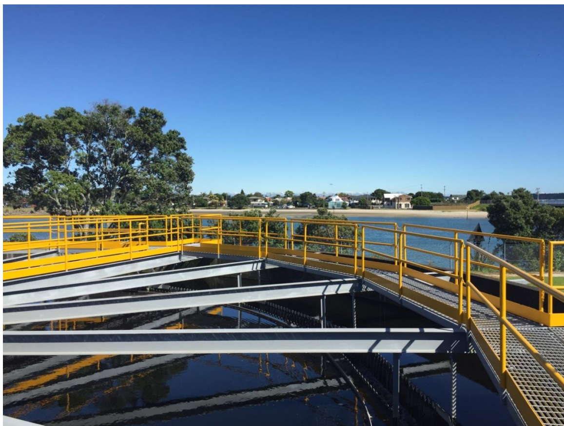
Figure 2: Chapel Street WWTP
