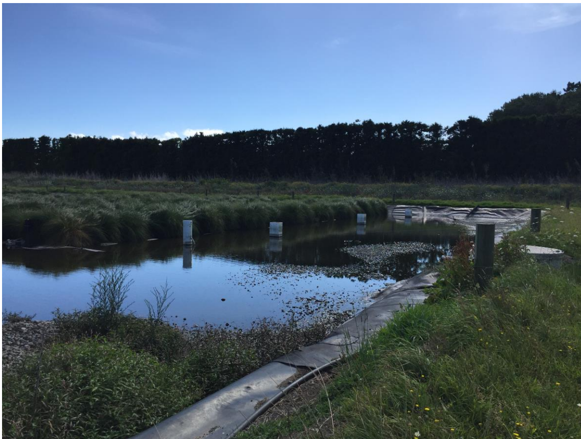
Figure 4: Floating wetlands at Katikati WWTP
