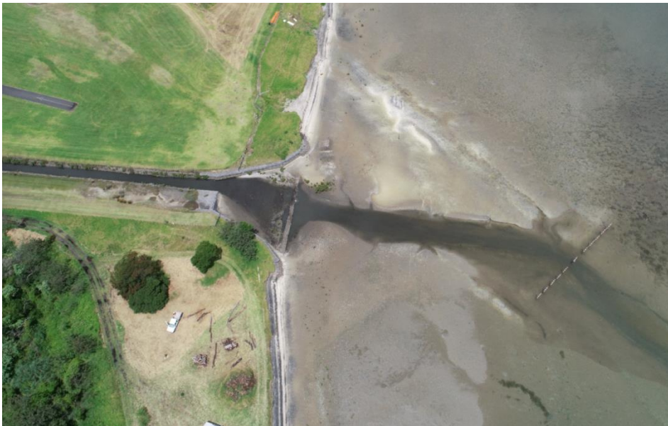
Figure 1: Discharge from the Airport Drain as photographed by BoPRC drone on 20 December 2018
