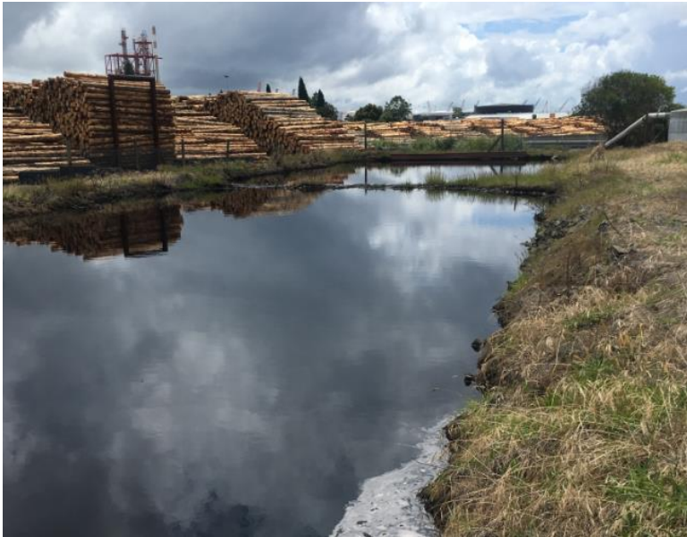
Figure 2: Port of Tauranga Hewlett's Road Log yard Stormwater settlement pond.
