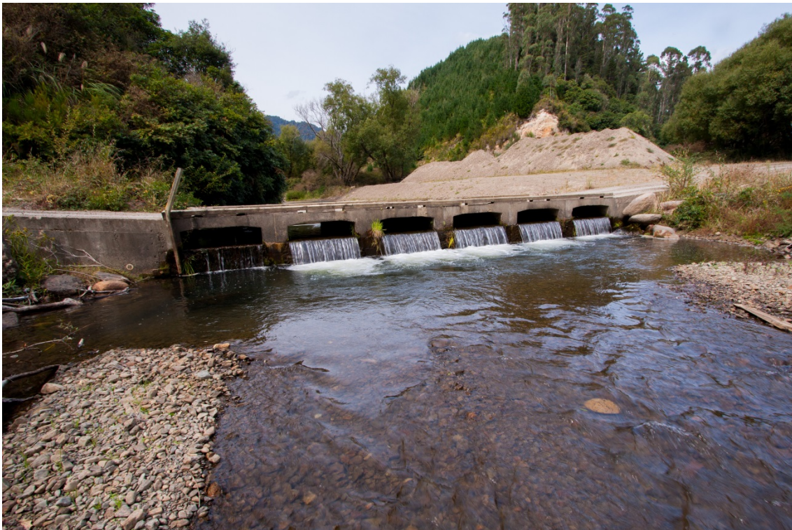
Figure 46 Example of a poorly designed road crossing that may act as a fish barrier, especially during low flows. However, such a structure may be beneficial if the stream above here is to be managed for either non-migratory species, or only for species that have good climbing abilities and which can surmount this obstacle. In this way, it may be possible to keep introduced species such as rainbow and brown trout from colonising new streams, if this is a desired outcome.
