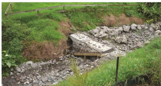
Works in stream beds such as building bridges or dams may need a consent
