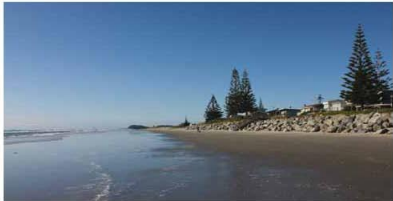
Coastal Protection works, Waiti Beach
