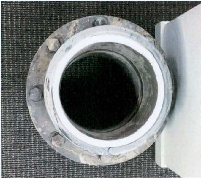
Figure 4-3: Photo of section of pipe
