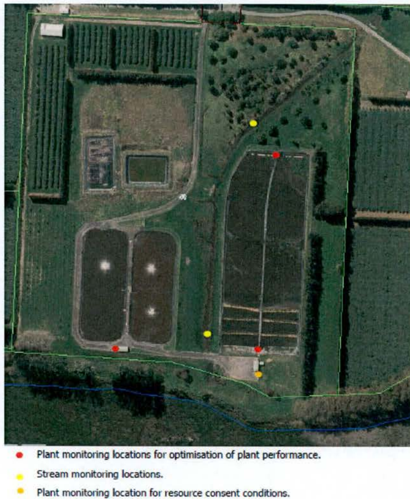
Figure 4-6: Monitoring locations at WWTP site
