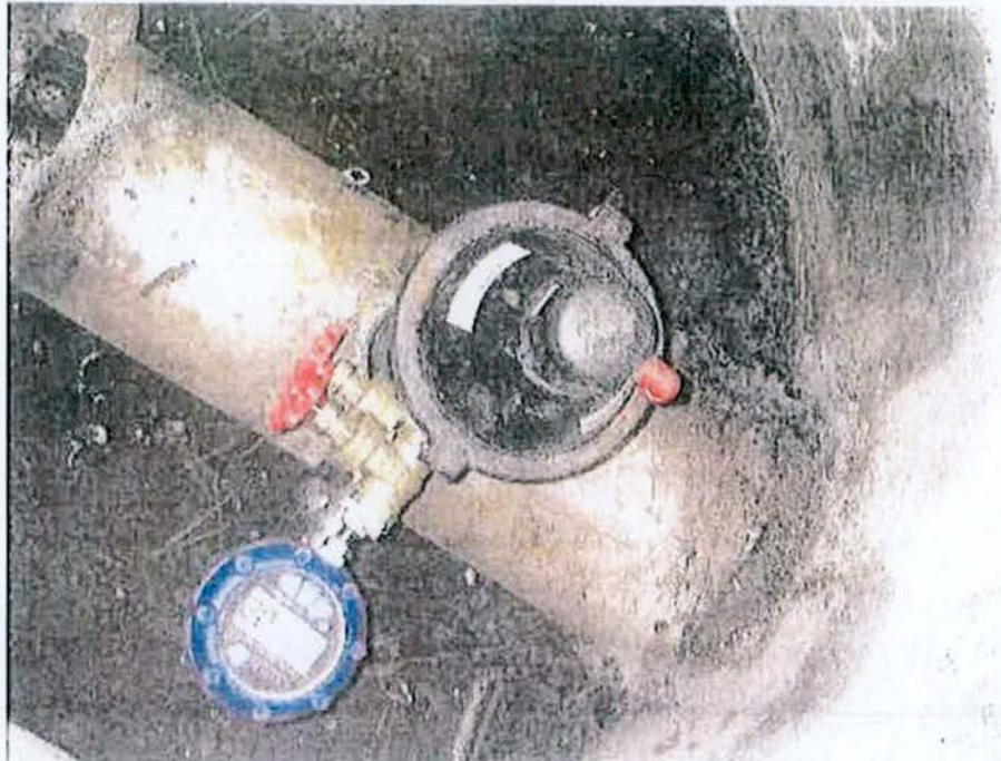
Plate 2.1: Dual dataloggers installed on air valve connection
