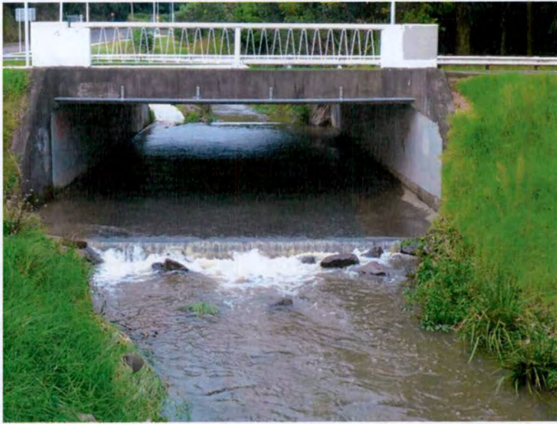
Photo A7: Wainui Te Whara Stream downstream of Valley Road during a small flood (18 April 2016).
