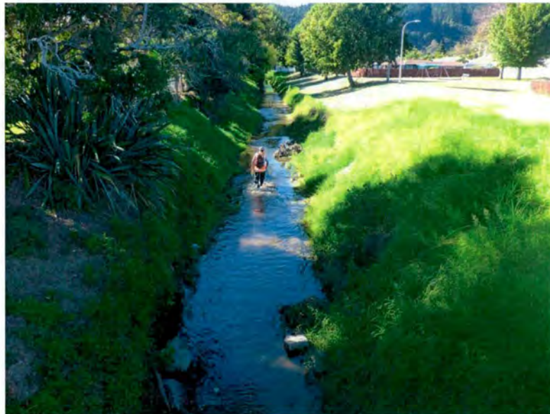
Photo A2: Wainui Te Whara Stream downstream of King Street (facing upstream 14 April 2016).
