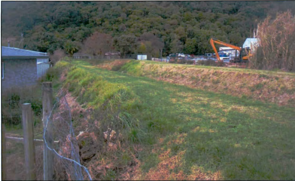
Figure 17: View east of Chainage 260- 360m.
