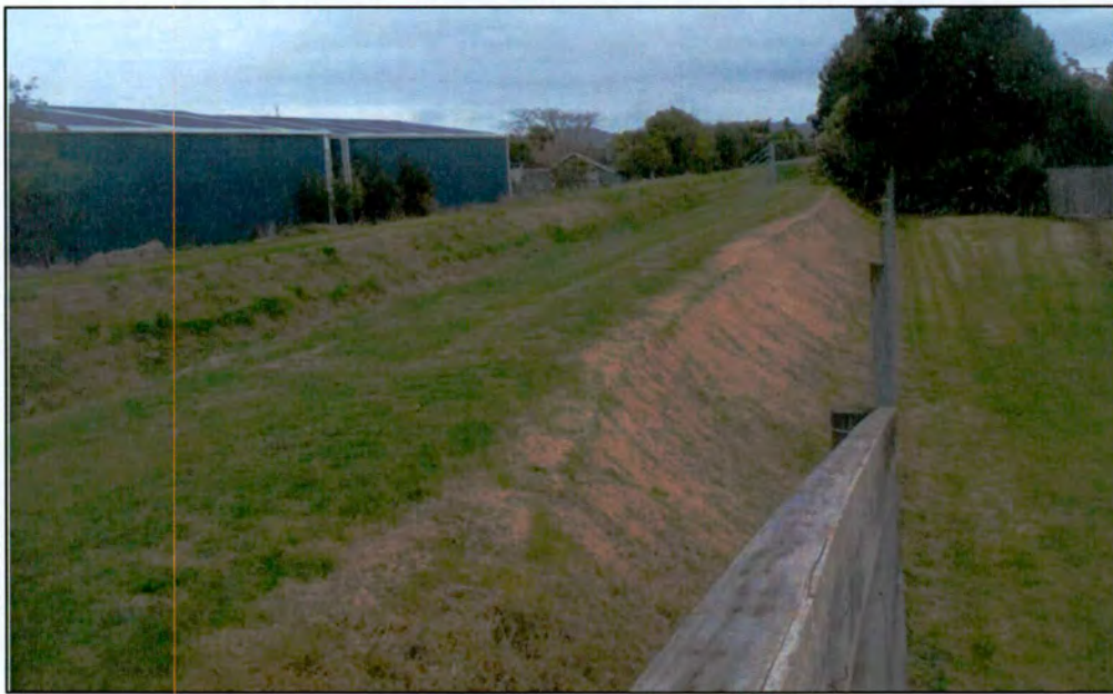
Figure 18: View west of Chainage 360-480m.
