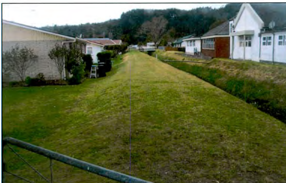
Figure 19: View east from King St of Chainage 900- 1100m – note the Baptist Church on the far right.
