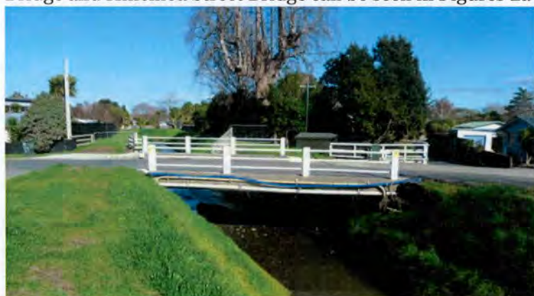
Figure 2a Douglas Street Bridge looking downstream
