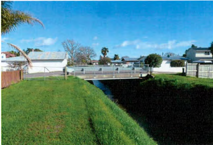
Figure 2b Peter Snell Street Bridge
