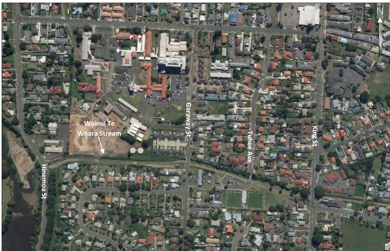
Figure 3: Aerial Photograph - Western Section
