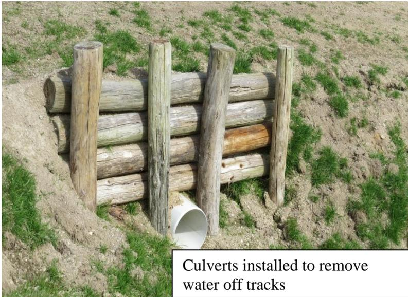
Culverts installed to remove water off tracks
