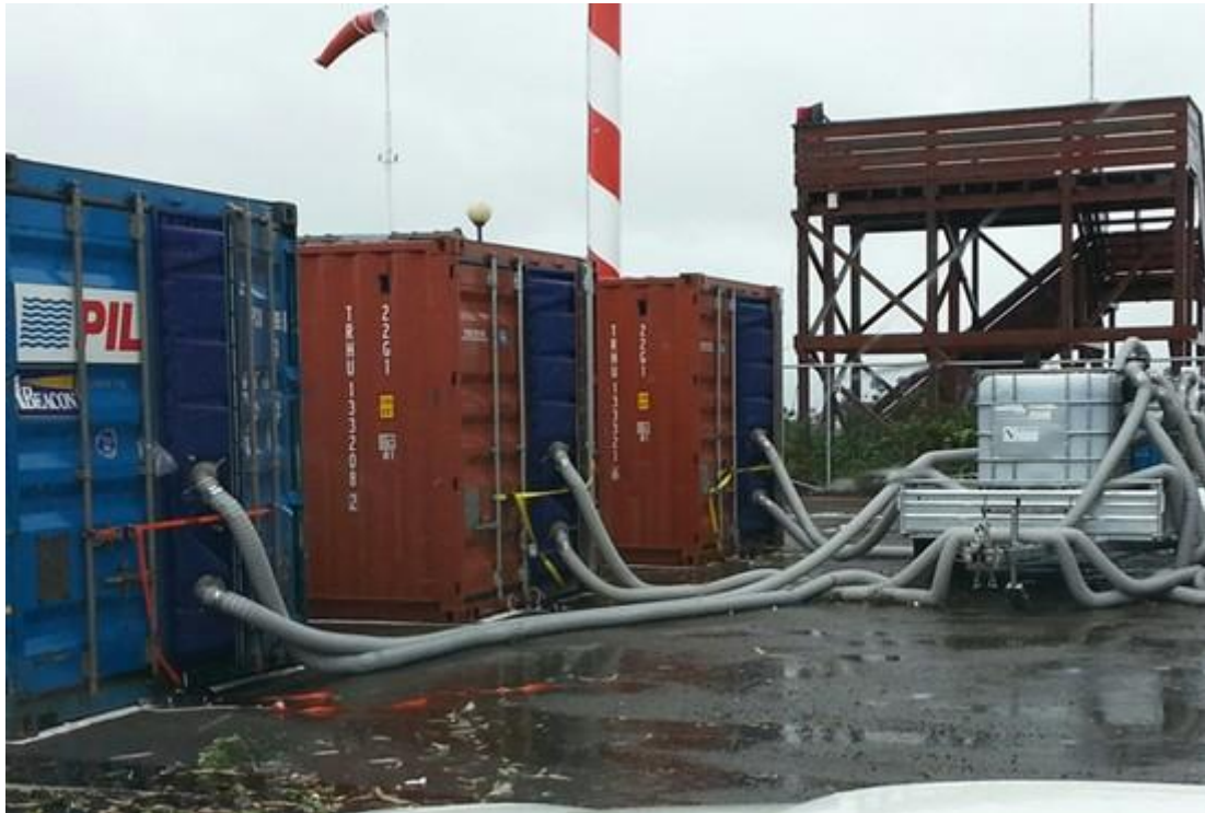
Photo: Recapture unit capable of capturing methyl bromide from 4 containers simultaneously [Source: Genera Ltd website]
