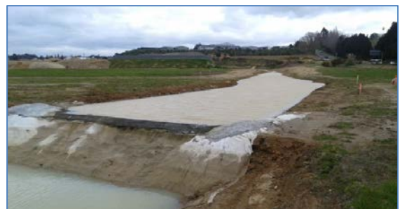
Image 2: A sediment control device, used to trap excess sediment draining from an earthworks site
