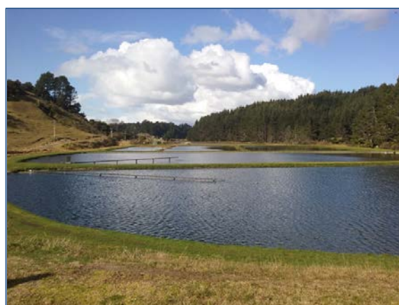
Figure 2: Ohope Wastewater Treatment Plant
