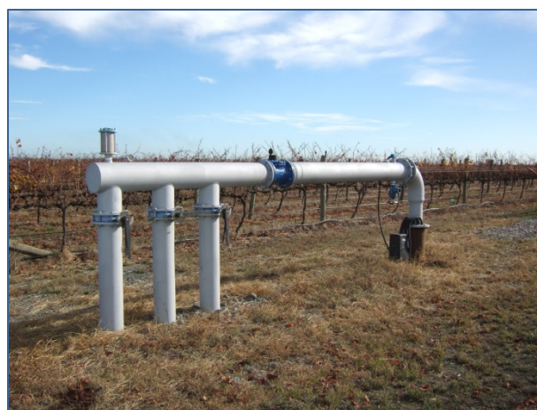
Image 18: A well configured groundwater abstraction bore, fitted with a water meter on the horizontal section of pipe.
