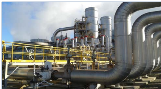
Image 16: The discharge stack from the Mighty River Power geothermal plant in Kawerau
