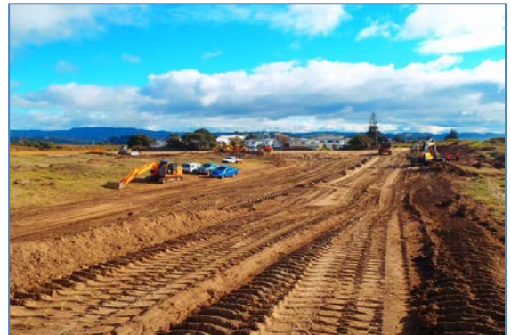
Image 1: Earthworks being undertaken for a residential subdivision in Ohope
