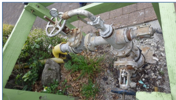
Image 14: A well-configured geothermal water bore in Rotorua
