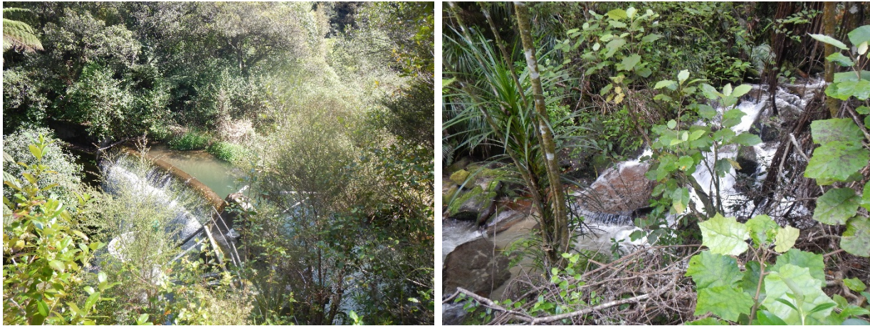
Figure 5: View of the dam spilling water, with the remnant flow spilling over the structure face (left). Rapid flows of the reaches below the dam (right).
