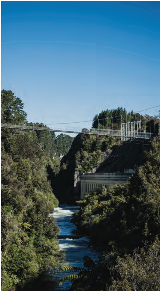
Arapuni Power Station on the Waikato River with Waikato River Trails Swingbridge
