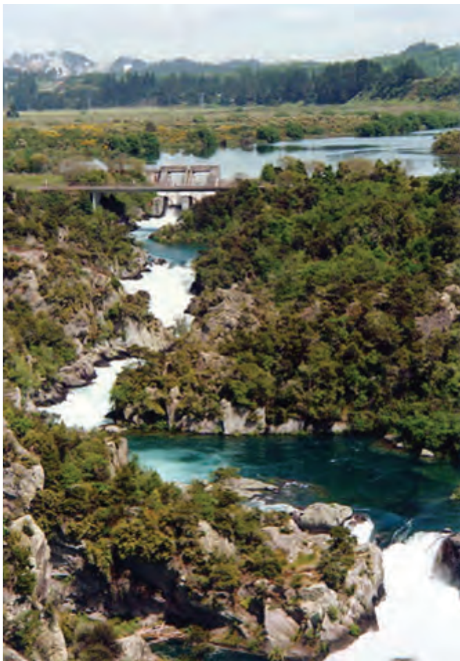
Heritage Shot - Waikato River. This photo gives some indication of how the Waikato River has changed with the advent of the hydro electricity system
