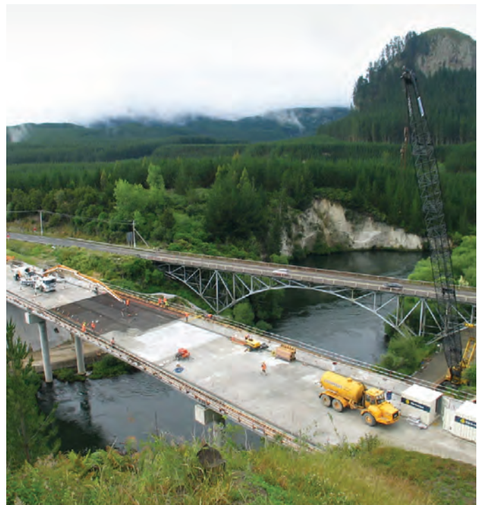
The new SH1 bridge at Atiamuri under construction in 2013. In partnership with NZ Transport Agency, Raukawa were heavily engaged in the project to replace the old bridge at Atiamuri
