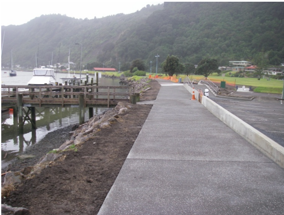
Figure 3.6 Concrete floodwall with access ramp, Muriwai Drive, Whakatāne.
