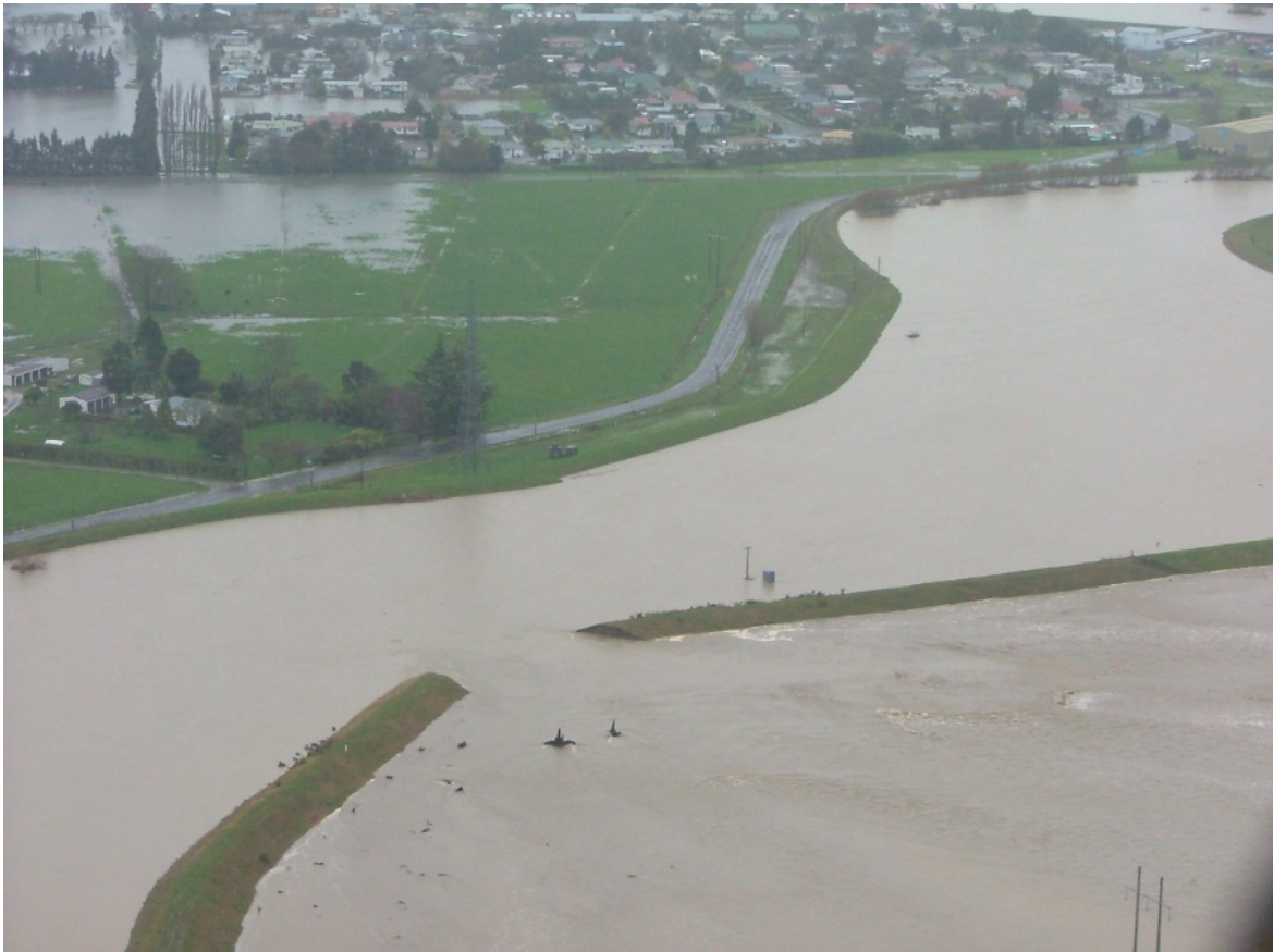
Figure 3.13 Stopbank failure at Sullivan's Bend caused by piping failure, Rangitāiki River.
