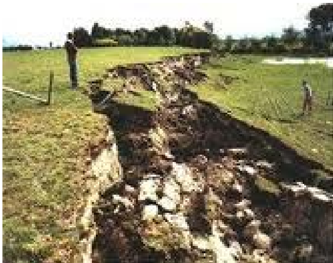
Figure 3.3 Stopbanks along Rangitāiki Plains showing lateral spreading damage to waterside shoulder resulting from 1987 Edgecumbe earthquake.
