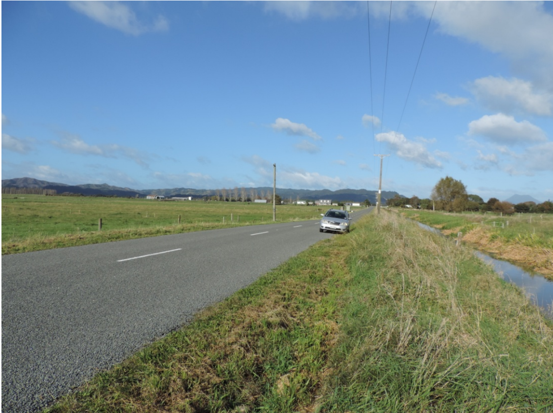
Figure 3.11 Sealed roadway/stopbank crest, Eastern Drain, Rangitāiki Plains.
