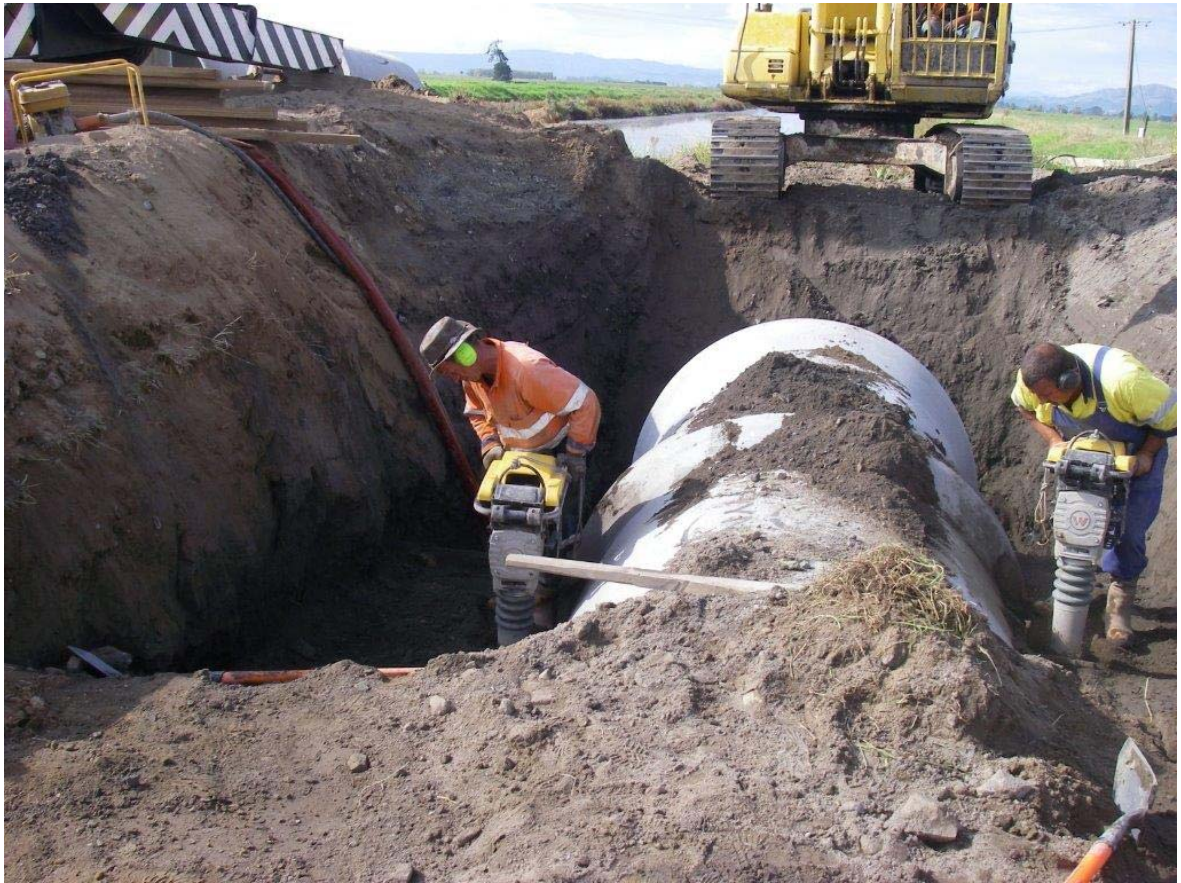
Figure 3.20 Example of well compacted drainage fill being placed around a culvert embedded within a stopbank.
