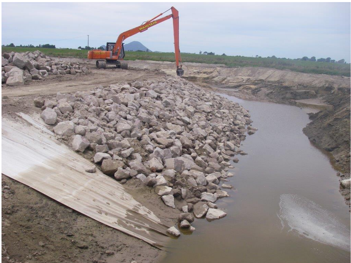
Figure 3.32 Riprap lined stopbank slope at Reid's Central Canal (viewing downstream).
