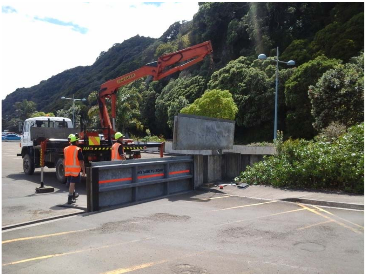
Figure 3.24 Installation of stoplogs within a stopbank system on the Whakatane River.
