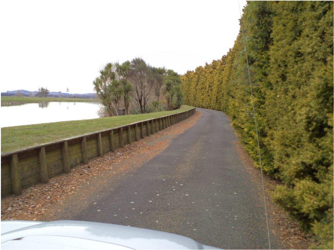
Figure 3.9 Partial timber flood retaining wall, Rangitāiki River.
