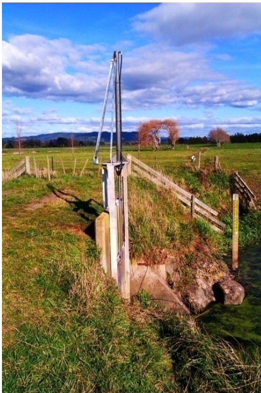
Figure 3.22 Hydraulic pack used to operate screw operated gates under hydraulic load.
