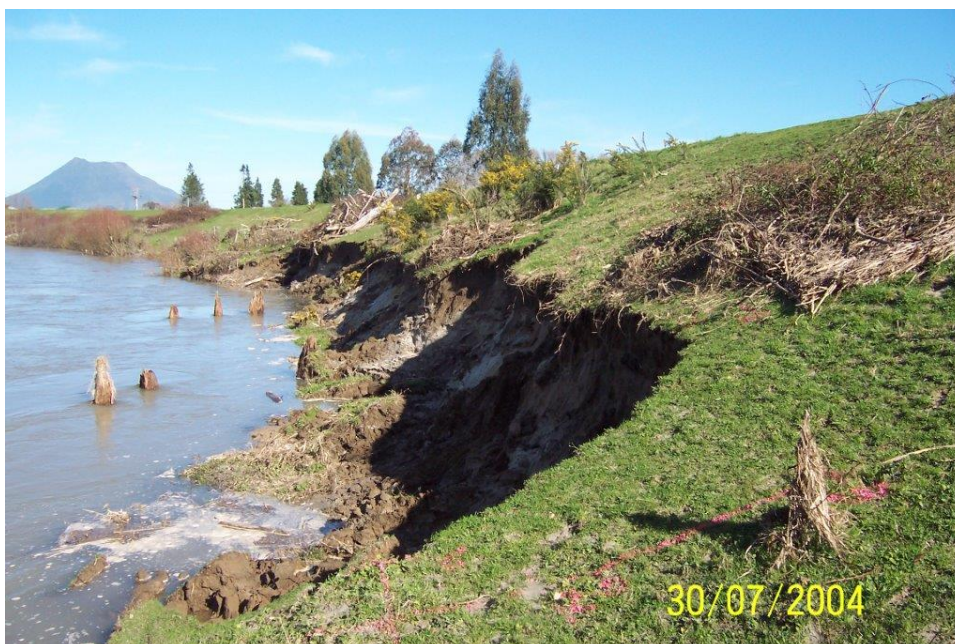
Figure 3.14 Undermining scour erosion, Pryor's stopbank, July 2004.
