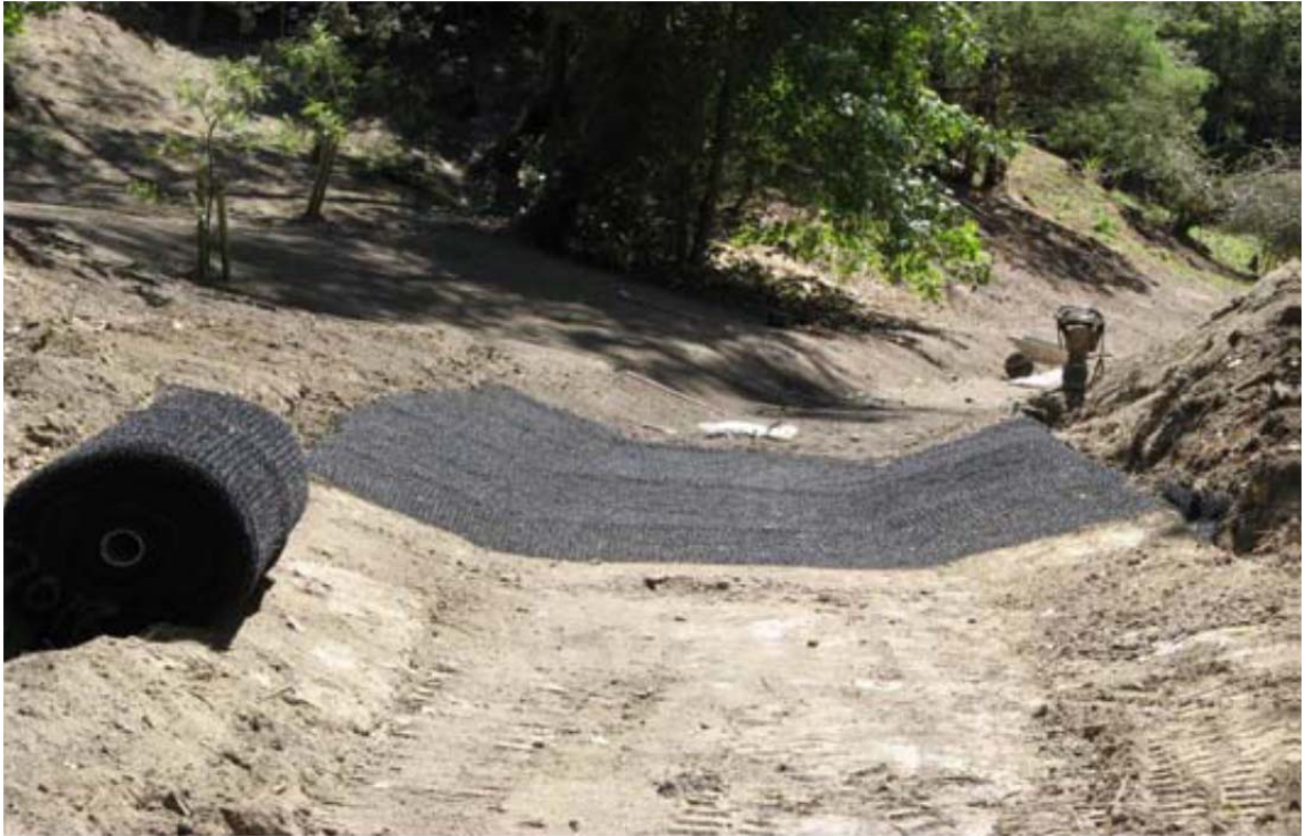
Figure 3.27 Maccaferri Enkamat, a geomesh, used to line banks of the School Stream, Havelock North, Hawkes Bay.
