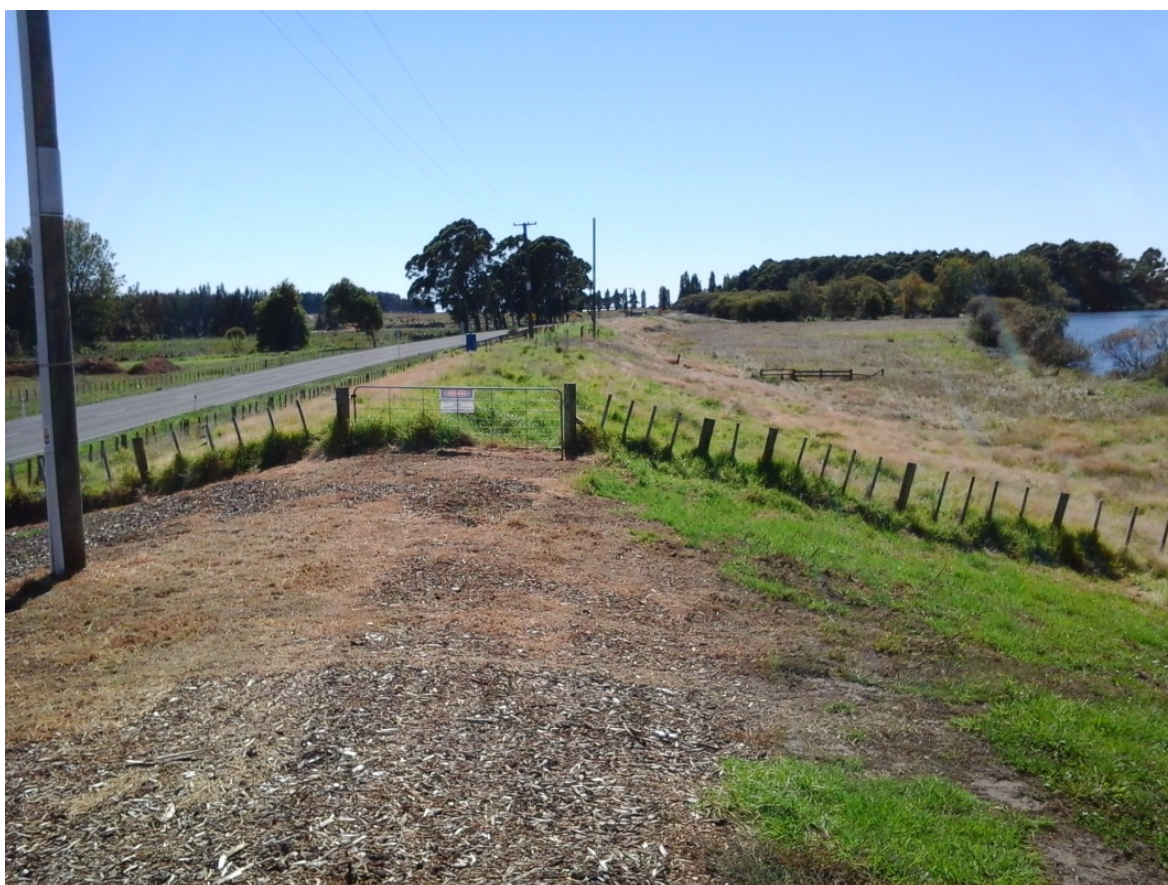
Figure 3.17 Fences around stopbank to protect grass cover from too much stock traffic, Kaituna River.
