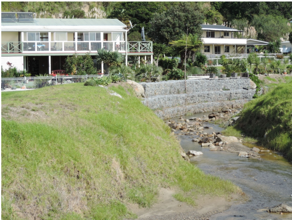
Figure 3.28 Maccaferri gabion baskets used to line and protect water side slope of stopbanks along the Awatarariki Stream, Matatā.
