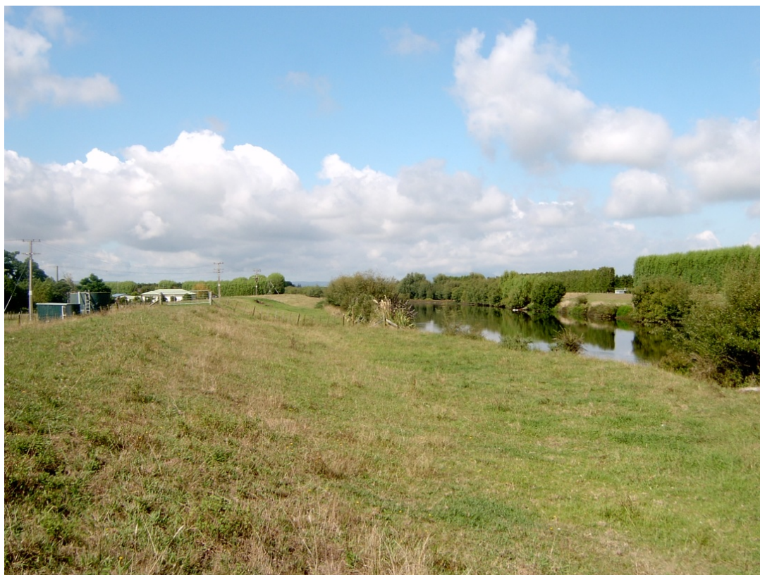
Figure 3.25 View of grassed slope of stopbank at Langdons Bend, Rangitāiki River (view upstream).
