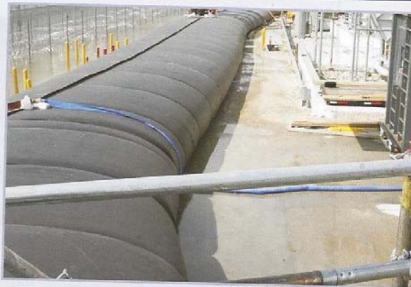
Figure 6.50 Water inflated barrier field setup (courtesy USACE)
