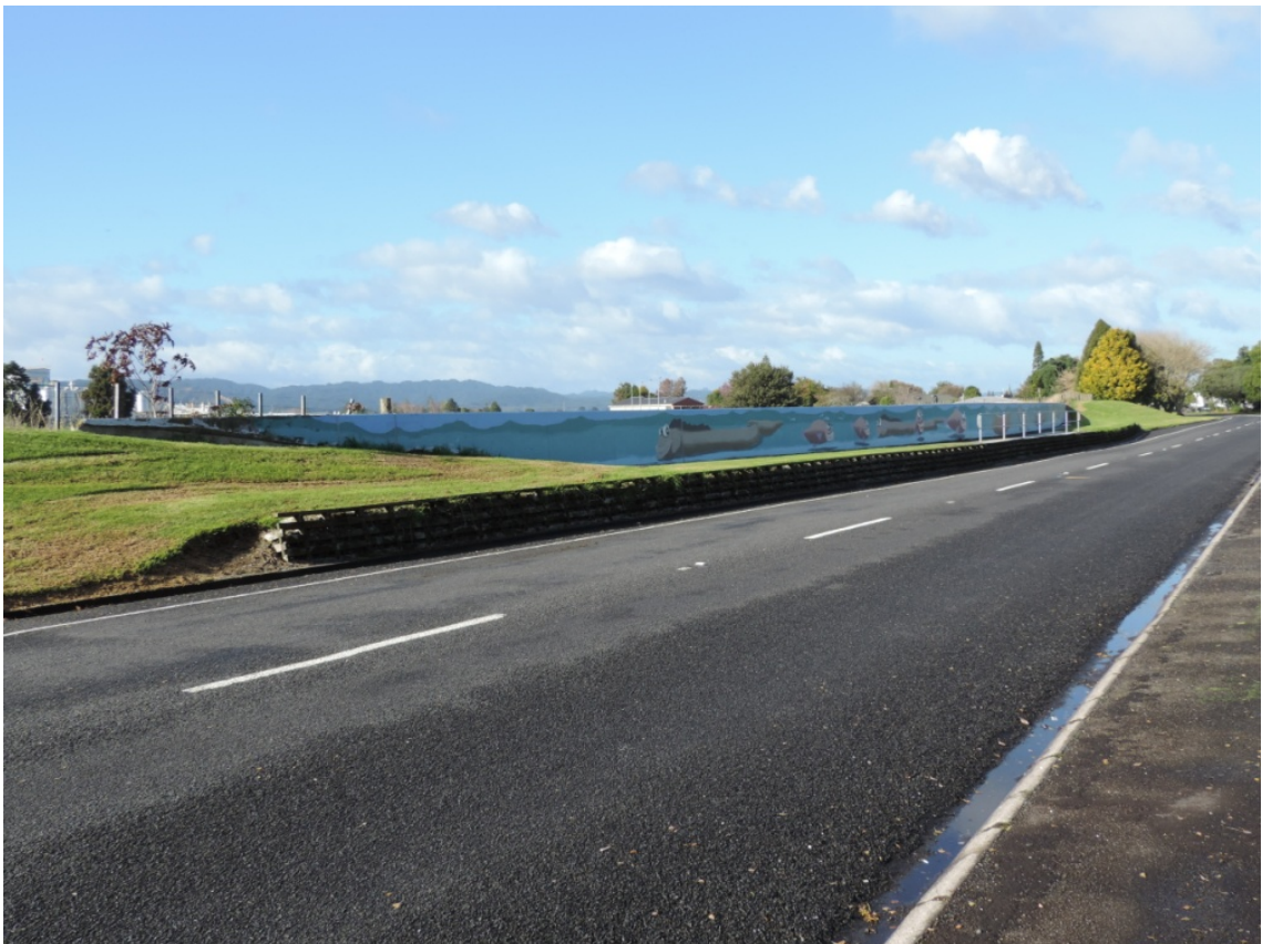
Figure 3.10 Part crib wall, flood wall and stopbank combination, Edgecumbe.
