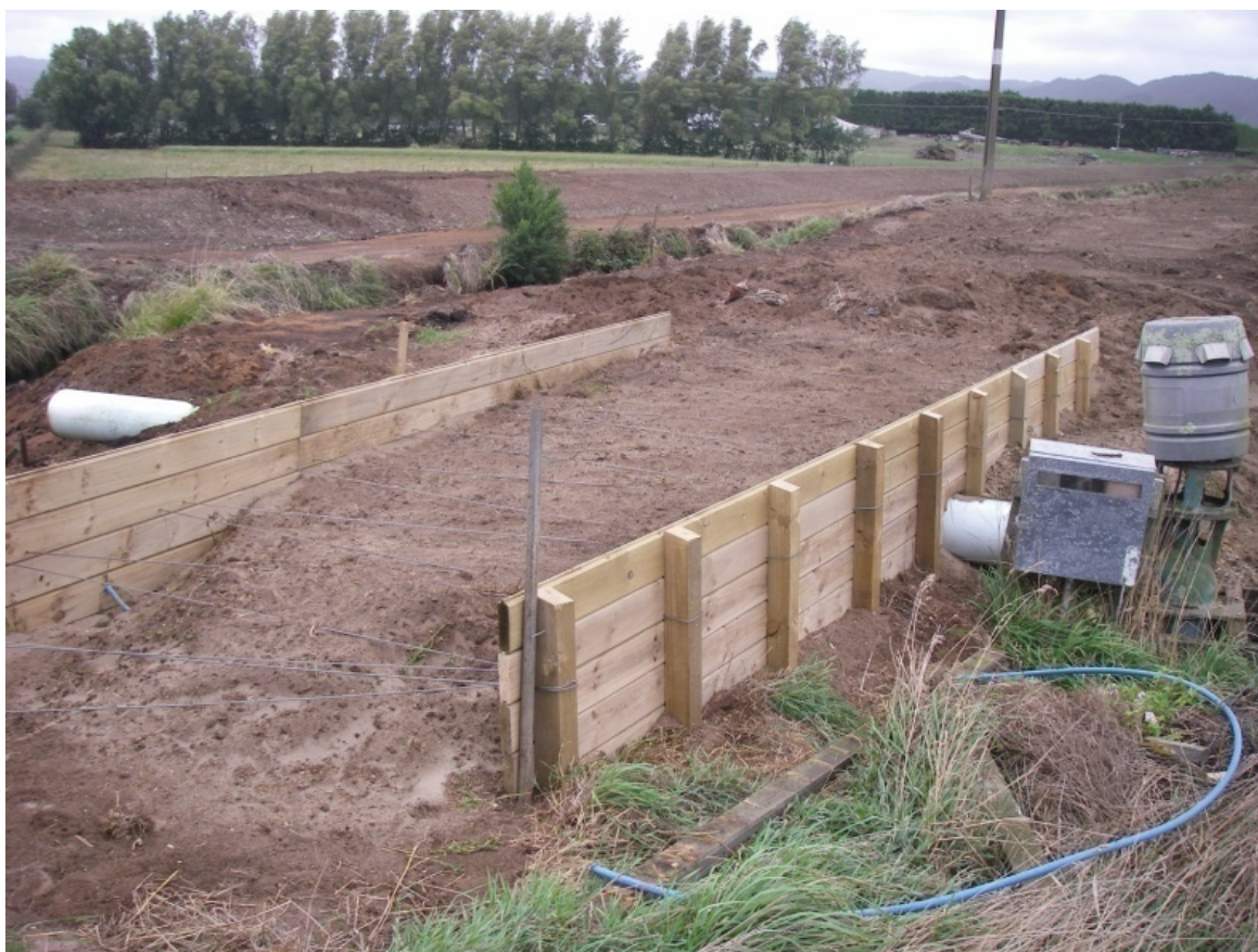
Figure 3.8 Full timber flood retaining wall showing pump pipework penetrating and tie back supports, Eastern Drain.
