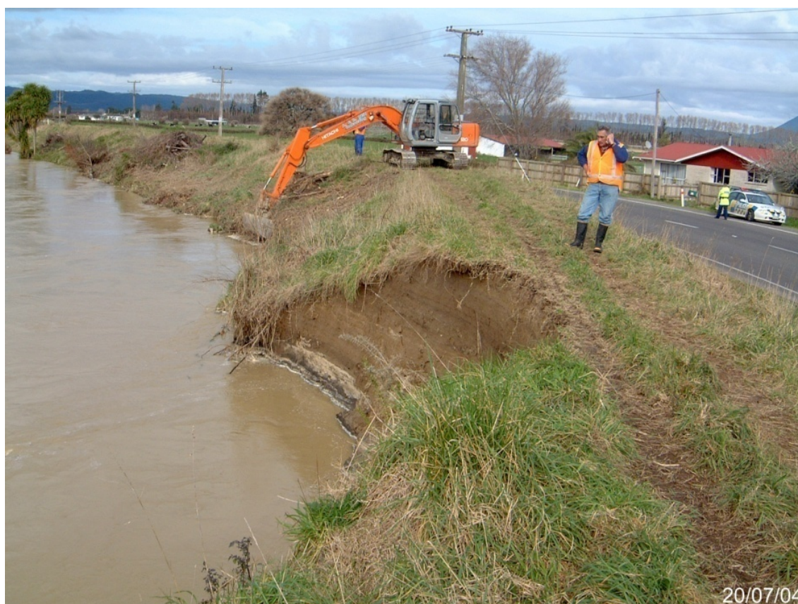
Figure 3.12 Collapse of the water side slope of a stopbank due to scouring, Kōkōhinau Bend, 2004.
