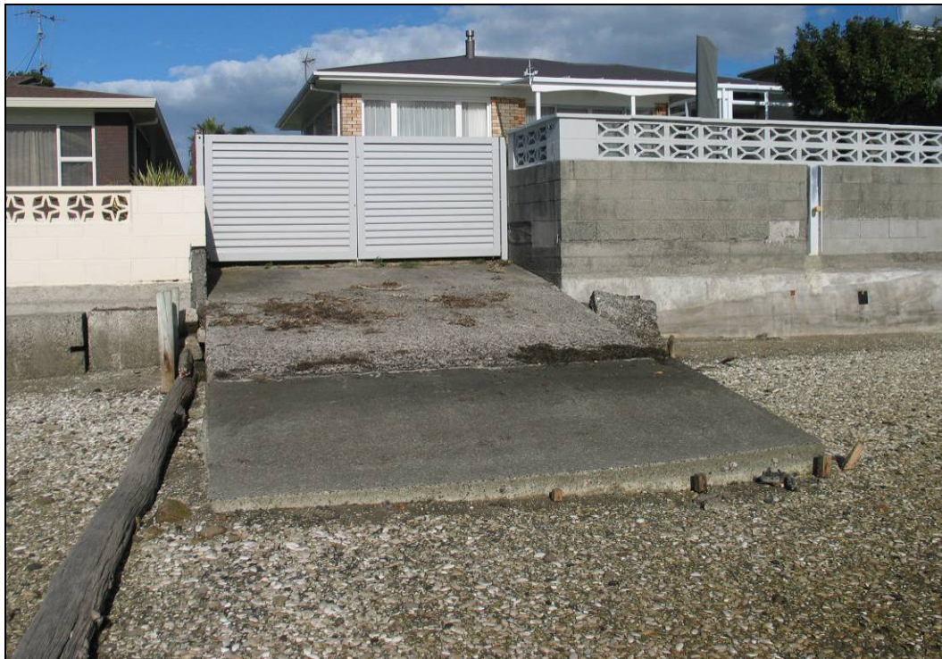
Figure 9. View of the concrete wall and slipway along the northern end of 11 Strange Grove where the storm water outlet is proposed.
