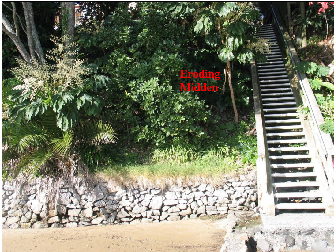
Figure 8. View of steps down coastal escarpment at northern end of Lot 15 DP 34289. Eroding shell midden is visible on the escarpment immediately adjacent to the steps and in the immediate vicinity of the proposed storm water pipe exit.
