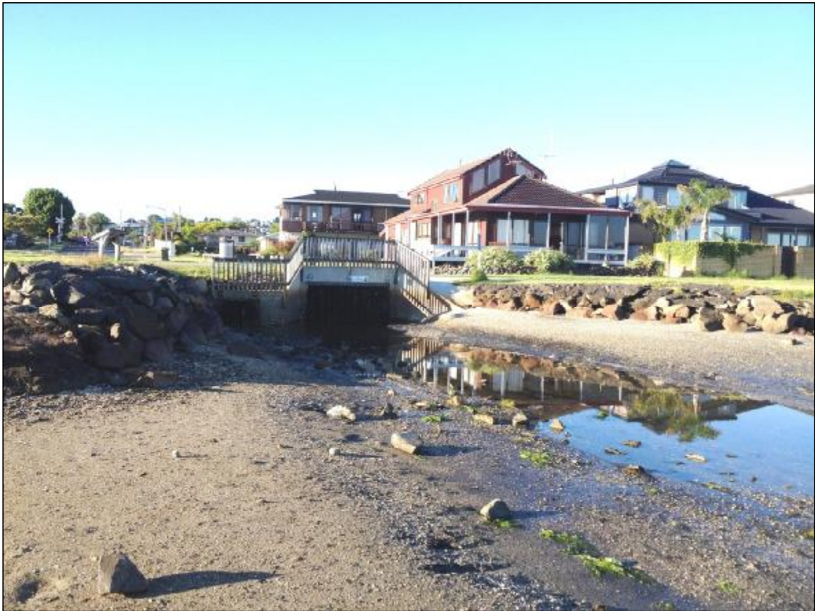
Figure 8-4: Stormwater Scour, Bureta Road
