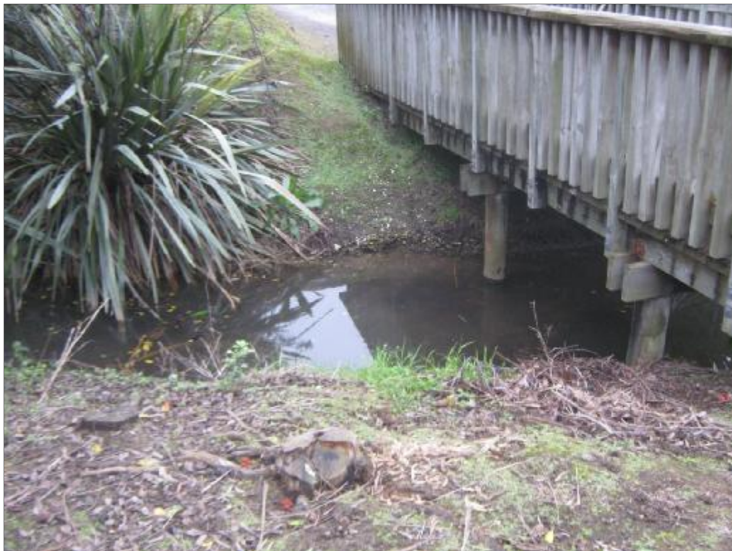
Figure 3-5: Sylvania Drive Open Culvert
