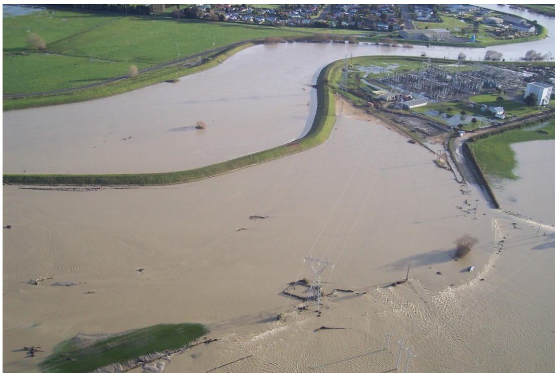
Figure 1.10 View of Rangitaiki River looking downstream at Edgecumbe with TransPower substation to right, July 2004.
