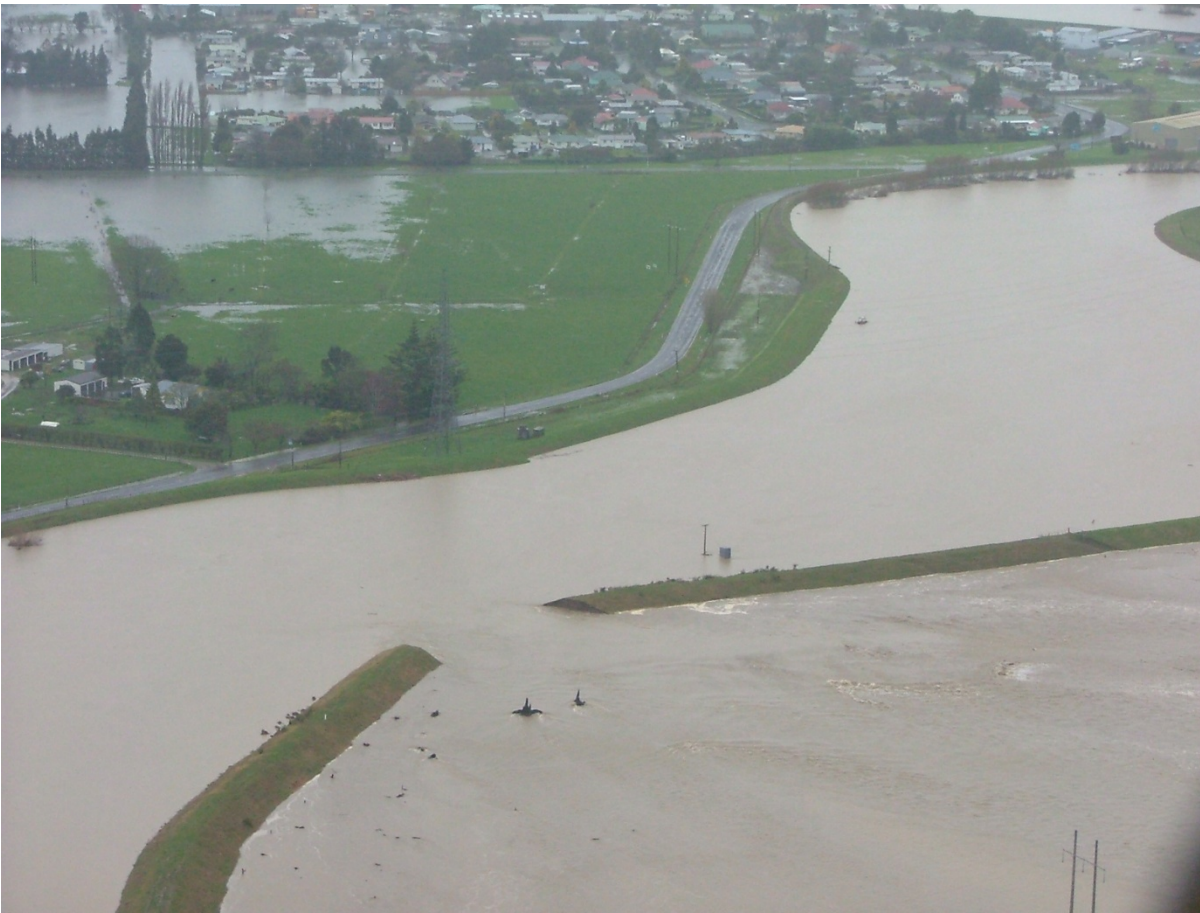
Figure 1.8 Stopbank breach at Sullivan's Bend, Rangitaiki River July 2004 (SW Edgecumbe in background).
