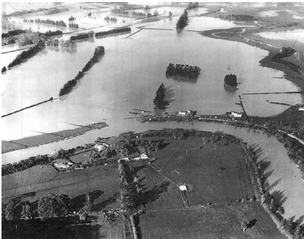
Figure 1.6 Stopbank breach at Reynolds Bend, Rangitaiki River in 1962 (river flow direction is from right to left in downstream direction).
