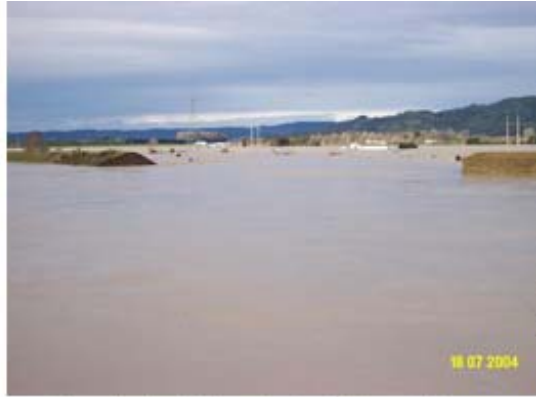
The stopbank breach by Sullivan's farm
