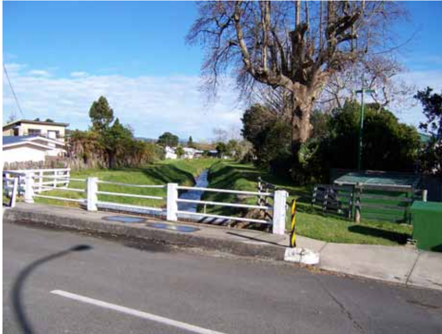
Figure 2.7 Downstream view of Wainui Te Whara Stream from Douglas Street Bridge
