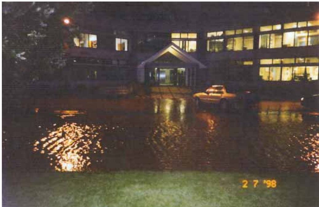
Figure 2.5 View of Environment Bay of Plenty's building showing flood waters in Quay Street during July 1998.
