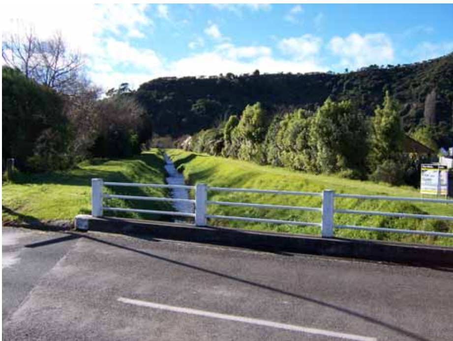
Figure 2.8 Upstream view of Wainui Te Whara Stream from Douglas Street Bridge
