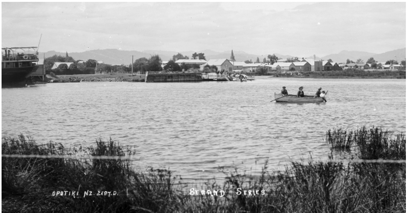
View of part of the Opotiki Wharf around 1910. Note the storage sheds and warehouses fronting onto the backwater in the distance, indicating the location of the earlier jetties. Alexander Turnbull Library, W A Price Collection G- 1310 1/2
