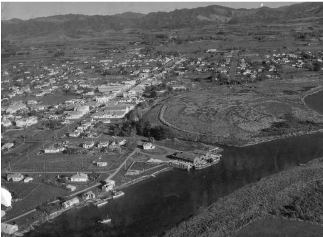
The wharf while still in its heyday, 1947, showing the triangular holding paddock with shelter shed, the loading race and wharf sheds. Further upstream on the Otara River were jetties, ramp, boatsheds and storage sheds belonging to Walker and Mokomoko. Savage's boatbuilding yards were also in this vicinity. The white building on the circular lawn was the Northern Steamship Co. office. Whites Aviation 7281 May 1947; Opotiki Museum Vol 3, 617
