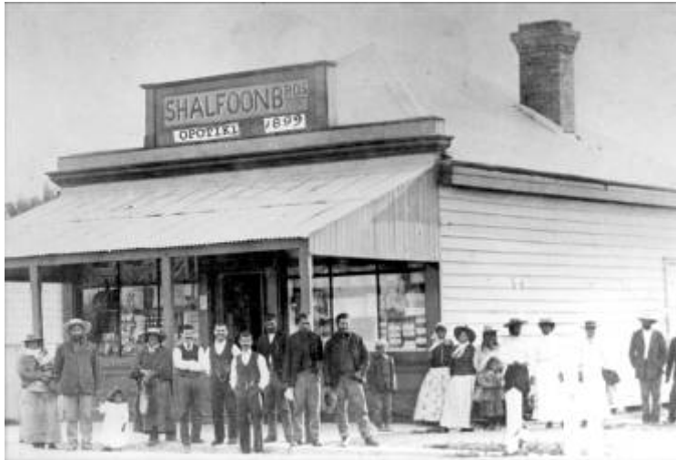
Shalfoon Bros Store on the corner of Kelly Street and Church Street is one of the earliest and most enduring family businesses in Opotiki. Opotiki District Council Photograph archive, Vol 2, 24.
