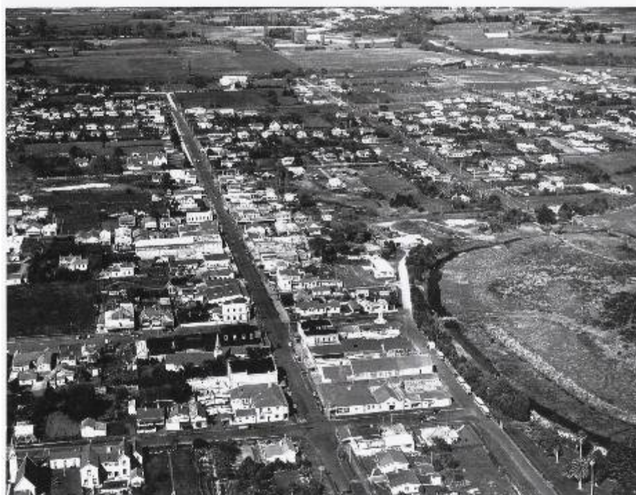
Aerial photo showing Church Street in 1951. The large two-storey building left foreground is the earlier convent. Whites Aviation 27663.
