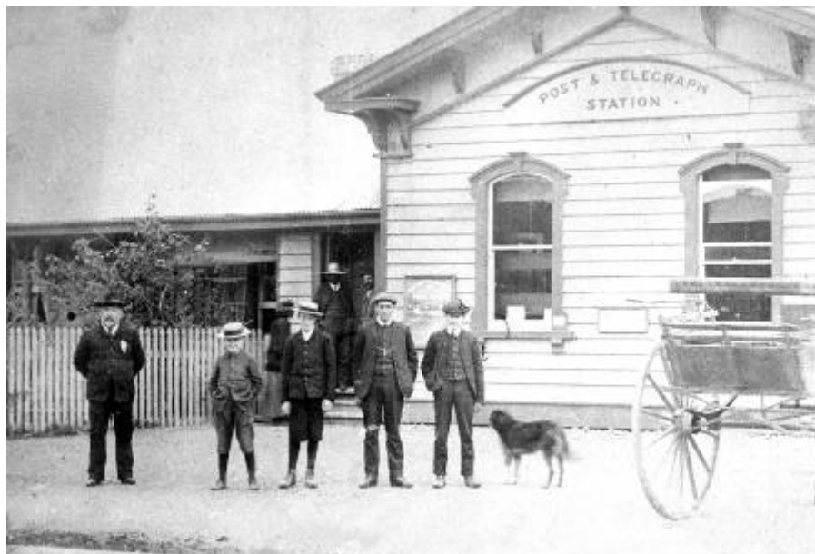
The first purpose built Post Office was built in 1874. After it burnt down in 1911 it was replaced by a larger plastered brick post office in 1913. Opotiki District Council Photograph Archive, Vol 1 156
