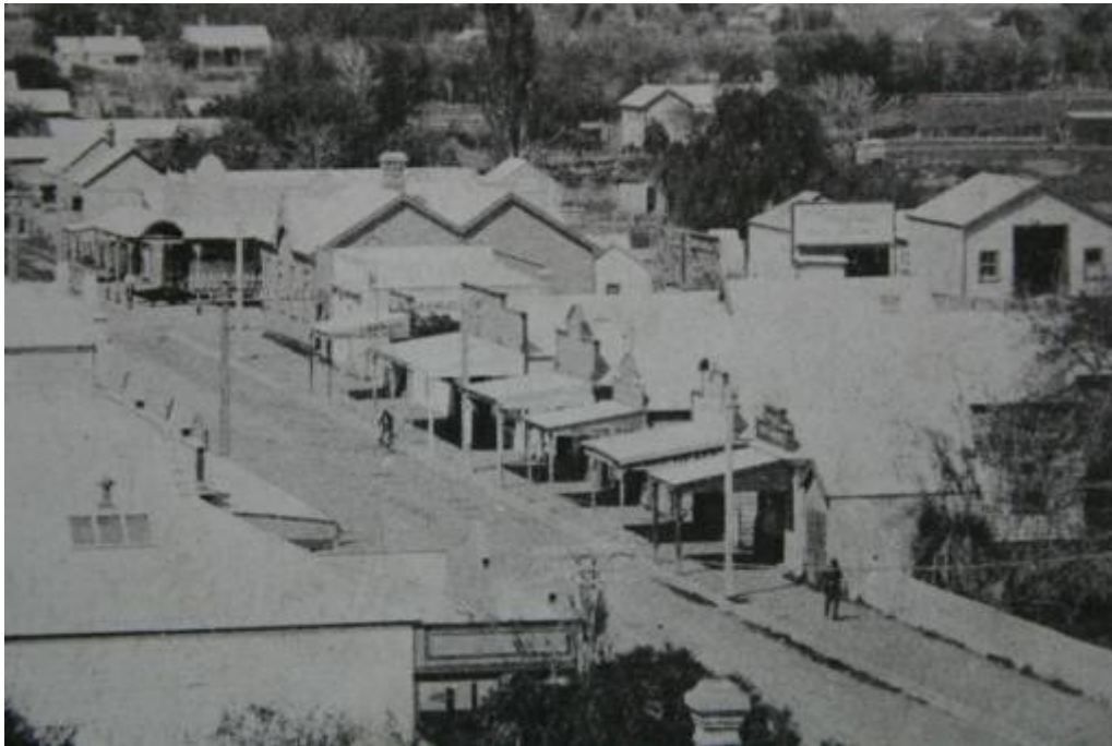
Early shops along Church Street were modest timber buildings with simple parapets. An exception is the larger two-gabled Mechanics Institute, the first library. It is partly obscured by a building believed to have been the Borough Council office in 1916. Close up of above photo, Vol 1, 170.
