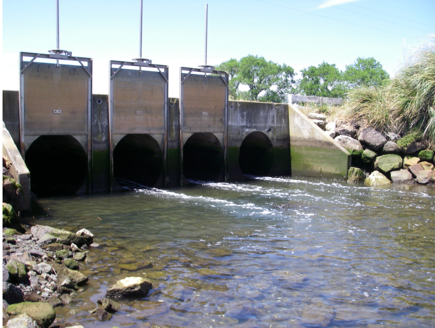
Figure 0-2 Fords Cut Culverts
