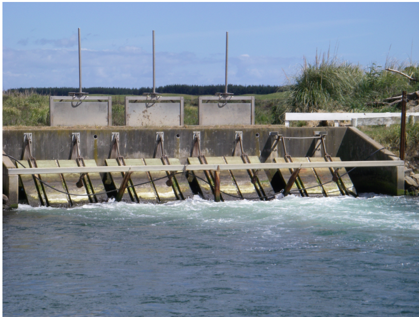
Figure 0-1 Fords Cut Tidal Gates
