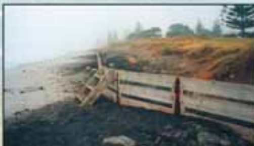
December 1998 The dilapidated and non-functional seawall Note erosion on the landward 'protected' side.
