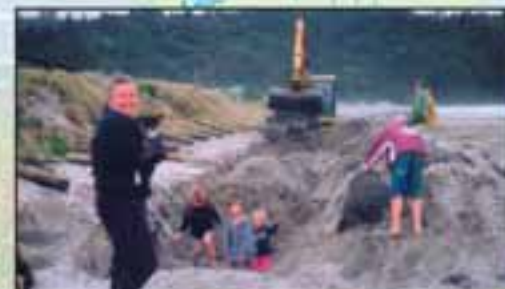
June 2003 All smiles as the removal progresses.
