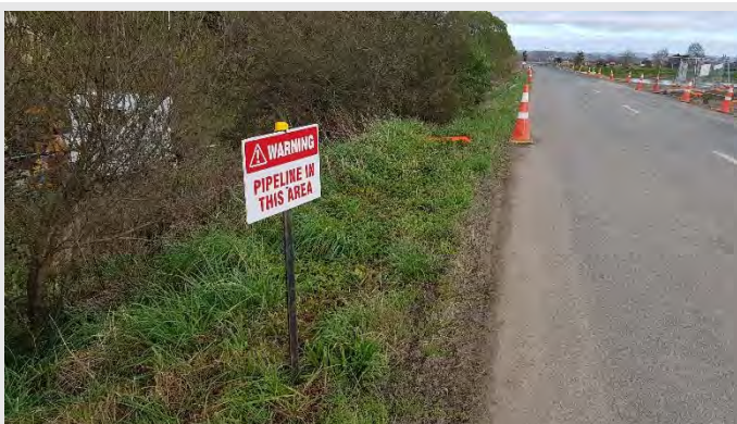
Photograph 16: Shoulder closure and warning signs for the sediment transfer pipeline along Shaw Road.
