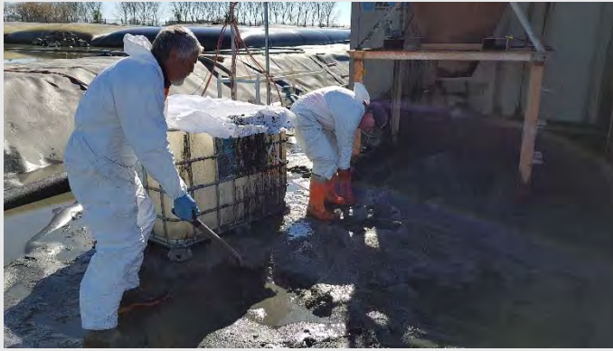
Photograph 13: Clean-up of sediment from within the CS1 water treatment area bund after an overflow due to dredging into heavy sands.
