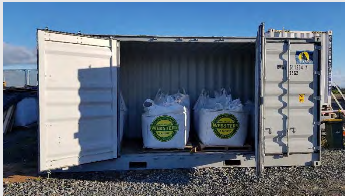
Photograph 10: Lime being stored at CS1 prior to being added to the sediment within the geobags.
