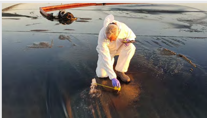
Photograph 12: Checks of the geobag damage and coordination with Geofabrics Limited as to the best methodology for repair.
