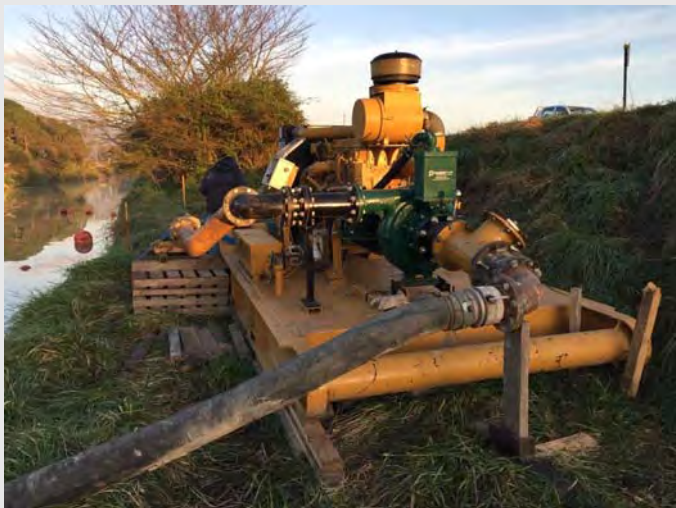
Photograph 21: New booster pump installed adjacent to Shaw Road.
