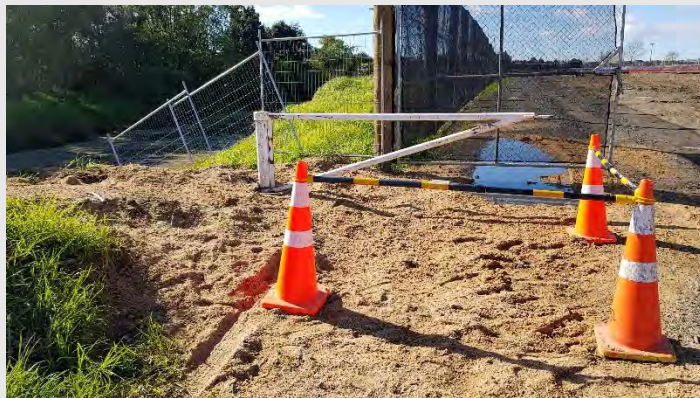
Photograph 6: Clean soil placed over the top of the potentially contaminated stopbank material disturbed during the gate installation.
