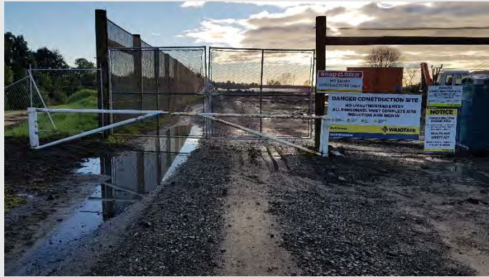
Photograph 5: New forestry gates installed at CS3 after a vehicle rammed the original gate.
