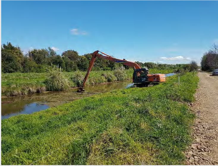
Photograph 22: Weed removal ahead of the barge.
