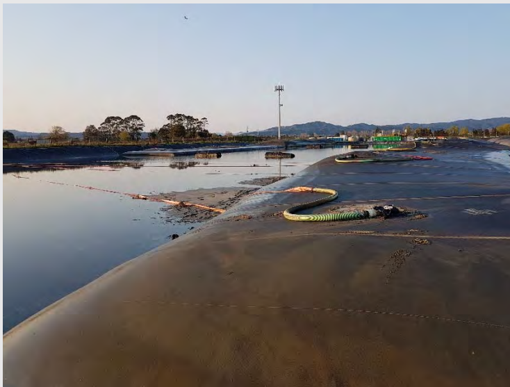
Photograph 11: Sediment spilled within the containment cell.
