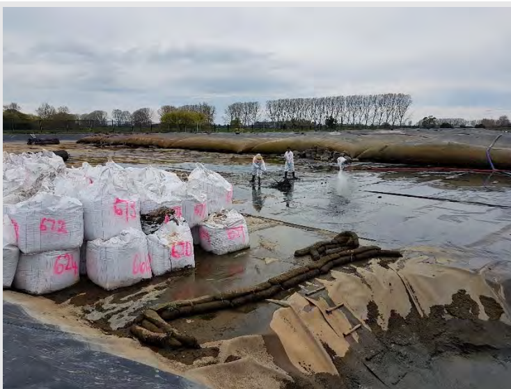
Photograph 15: Cleaning of the containment cell CS1 begins.
