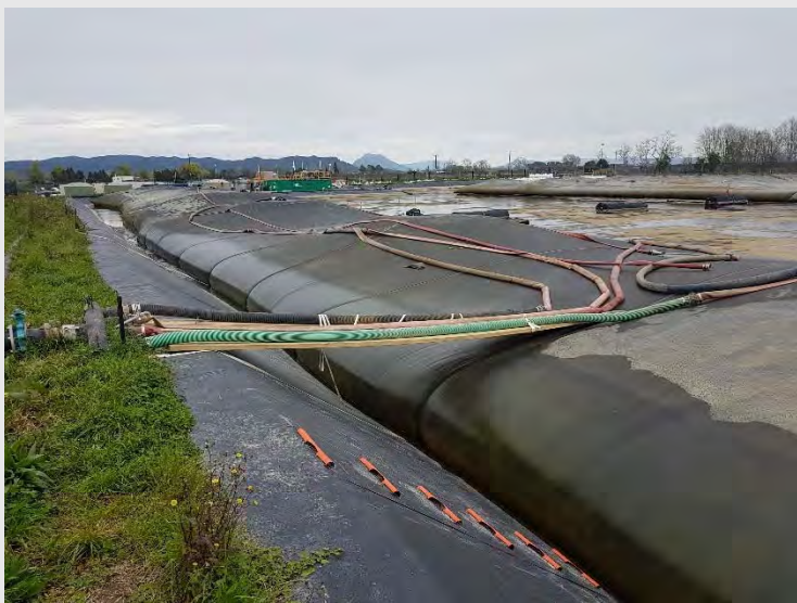
Photograph 12: Sediment transfer pipelines laid on wooden planks to reduce wear on the pipes.
