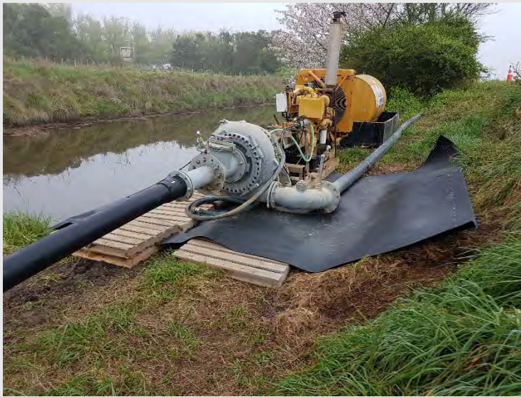
Photograph 13: Boost pump set up with HDPE liner to ensure any leakages return to the canal.
