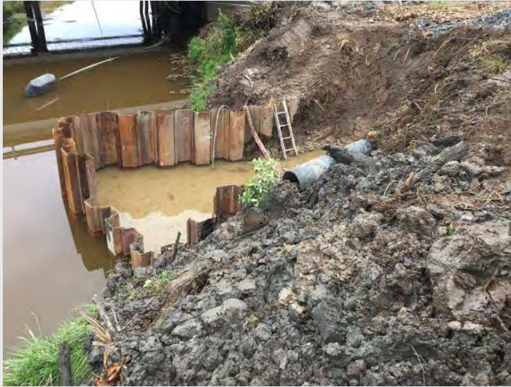
Photograph 4: Sheet pile installed for thrusting of a culvert under Shaw Road.
