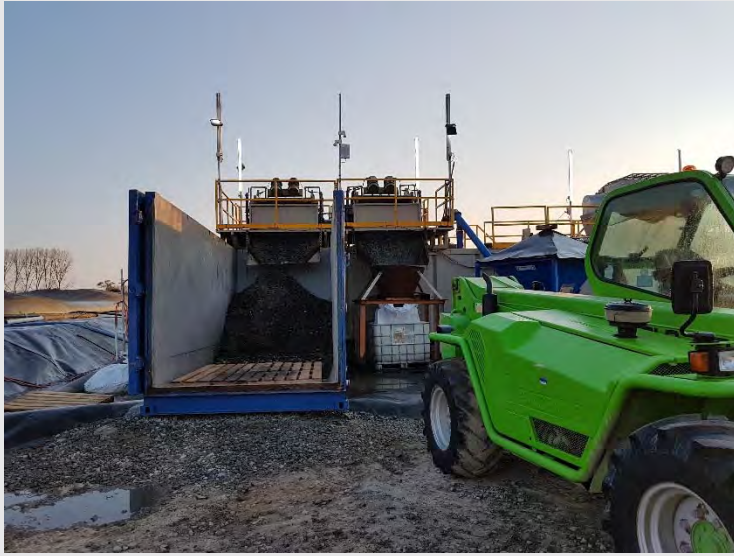
Photograph 10: New oversized material overflow bin set up.
