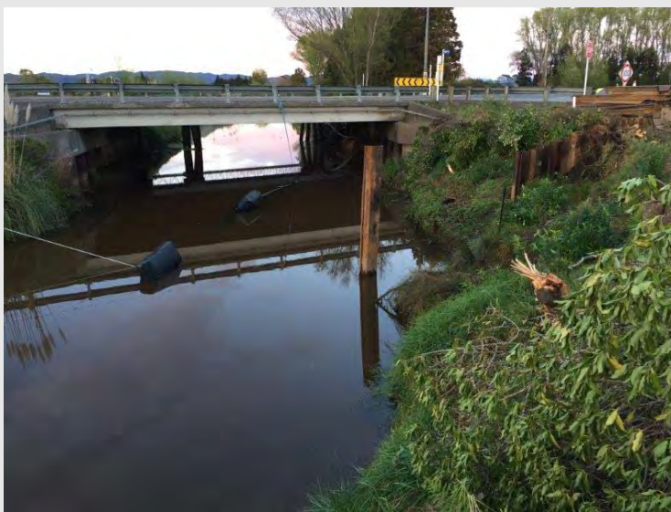
Photograph 6: Sediment transfer pipeline is floated past the newly installed temporary sheet pile.
