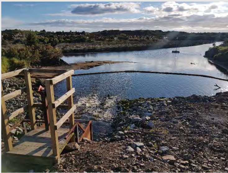
Photograph 23: FCS-East releasing water from the project area.
