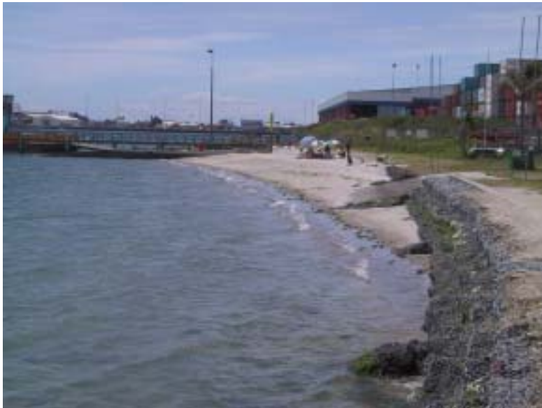
Diagram 6.7: Example of beach nourishment with partially buried gabion revetment.
