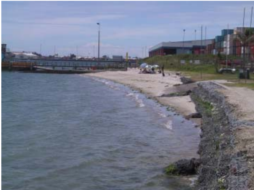
Photo 6.2.2. Sulphur Point (northern-end beach) after recent nourishment with 200m 3 of sand in December 2001. Due to site conditions nourishment here is required every 1-2 years.
