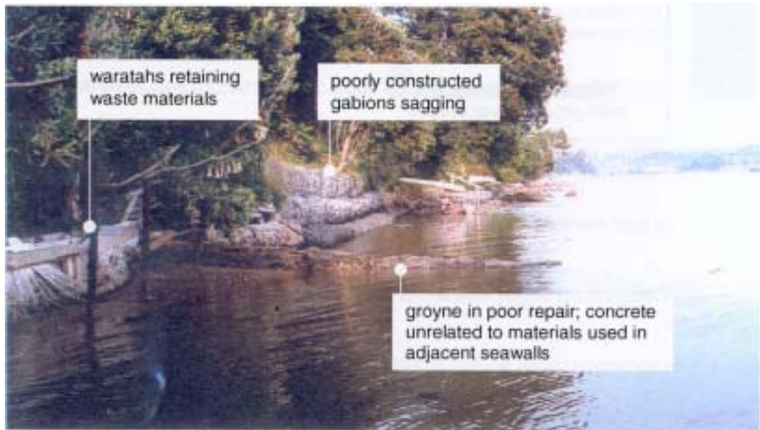
Figure 4.4 This photo shows a number of design and construction faults that make the area of harbour margin look unappealing and are ineffective.
