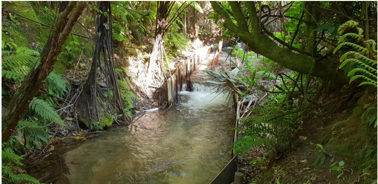
Figure 3: View upstream over the area of proposed works (looking toward the culvert outlet), illustrating stream incising and erosion. Protective boards have been installed as a temporary measure to reduce bank erosion.
