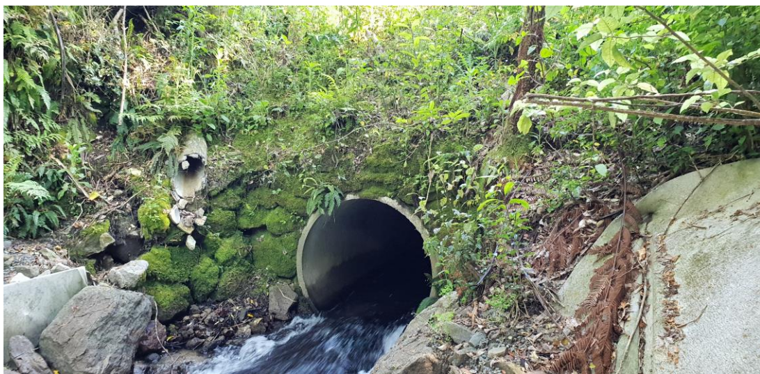
Figure 2: Current culvert outlet (installed approximately 30 years ago), at the northern end of the proposed stream works.
