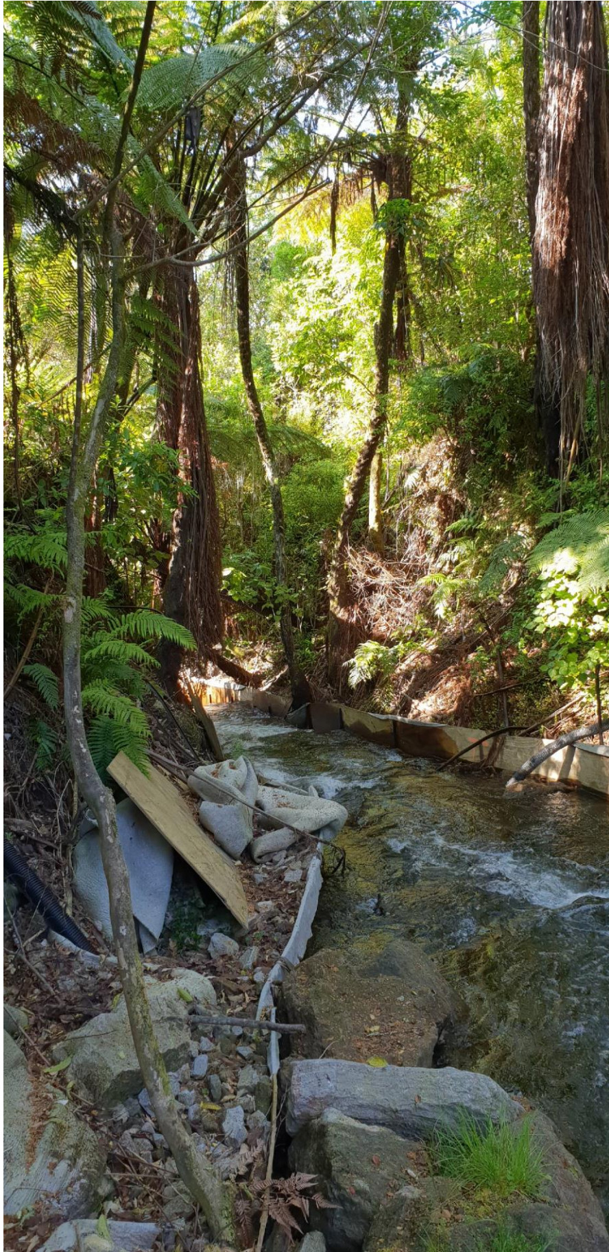
Figure 4: View downstream within area of proposed works (looking toward Lake Tarawera) illustrating current erosion and previous modification.
