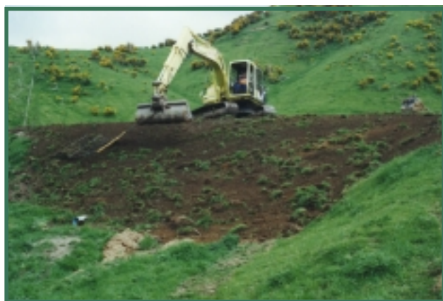
Use of chain harrows to mix seed into topsoil spread on a dam embankment. Harrows are being dragged by excavator arm
