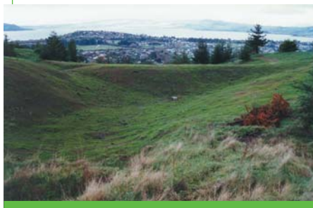
Completed dam; spillway is at left of embankment. Pipe intake can be seen at base of embankment.
