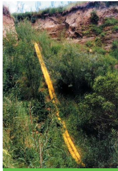
Flexible pipe flume (twin 160mm novacoil) carrying flow from a detention dam to the lower channel level.
