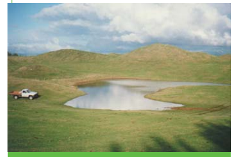
Impounded stormwater in a detention dam. Dams take 12-24 hours to drain depending on volume of water and flow rate of the outlet pipe. Embankment is at centre left of photo and truck is parked in dam spillway.
