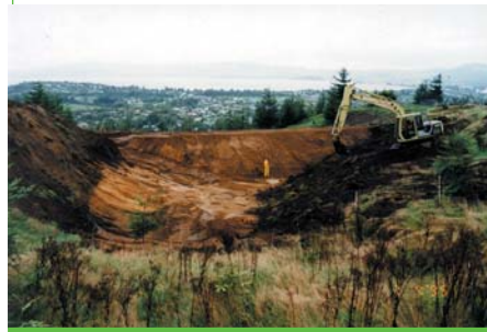
Detention dam under construction, topsoil being spread prior to sowing grass seed
