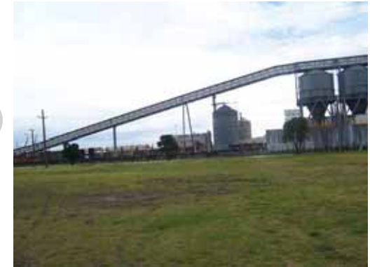
Conveyer to silos
