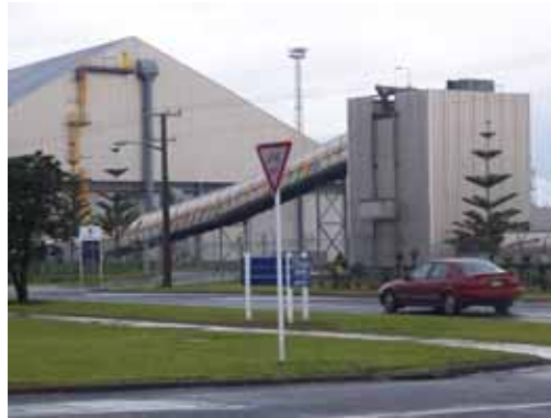
Conveyer from shed
