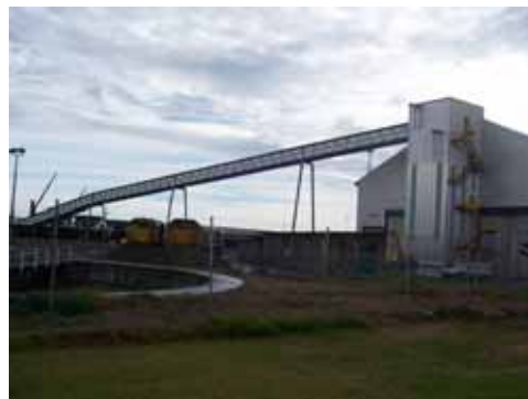
Conveyer to shed
