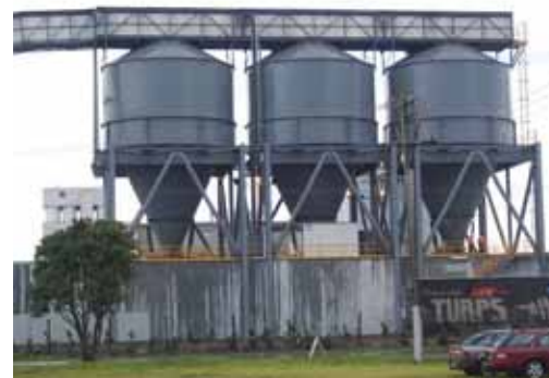
Silos discharge to train carriages
