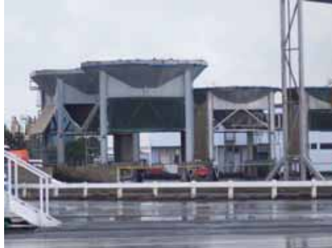
Grabs discharge into hoppers then into trucks
