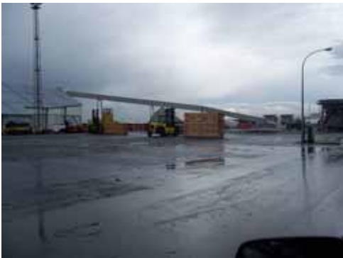
Conveyer to shed
