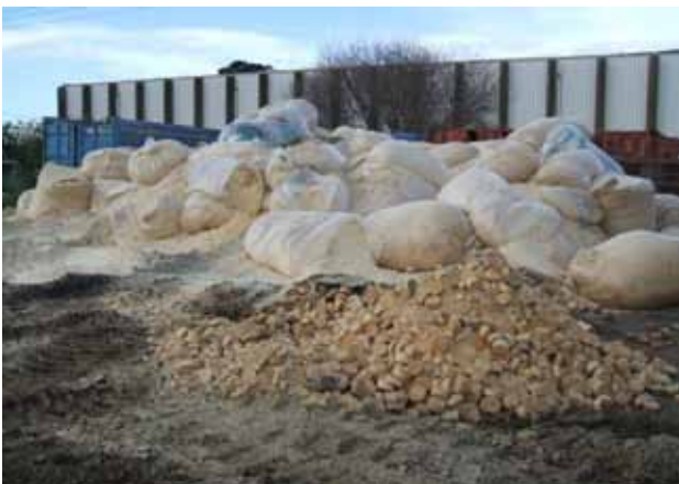
(Above) uncovered work areas like this result in polluted run-off and dust problems
