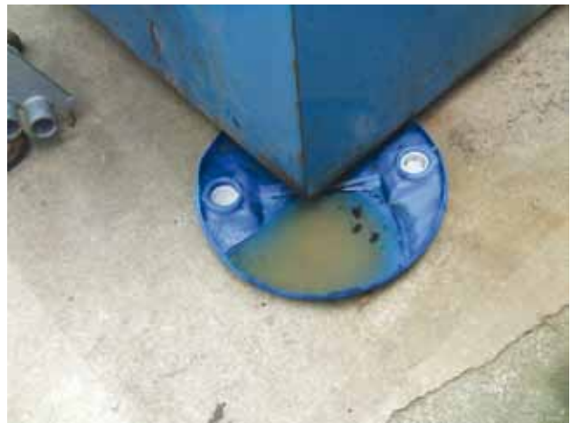
(Above) a waste skip for storing scrap metal is leaking oily water. Scrap metal bins should have lids to prevent rainwater entering them.
