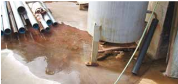
(Above) boiler blow down is directed to hardstand where it flows into a stormwater drain. This should be connected to sewer (with consent from Council).
