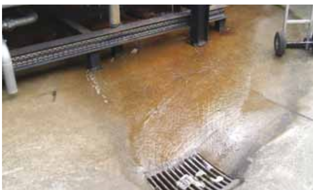
(Above) cooling system wastewater flows directly to stormwater. This presents a health risk to Council staff working on the network and an environmental risk to aquatic life. This should be plumbed to sewer (with consent from Council).
