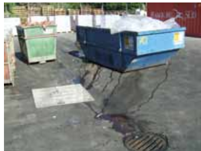
skips of waste are set out ready for loading on a hardstand with no bunding resulting in pollution entering stormwater drains.
