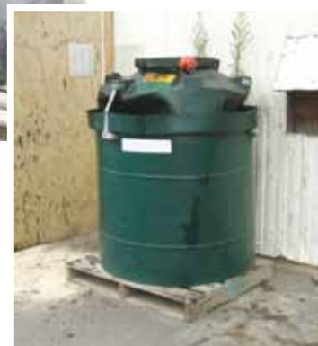
(Above) a number of spillages have occurred when filling this waste oil igloo. Contaminants will be washed away to stormwater when it rains. Ideally tanks should have a piped line for filling from the workshop or at a minimum a funnel should be used. This tank should also be covered.
