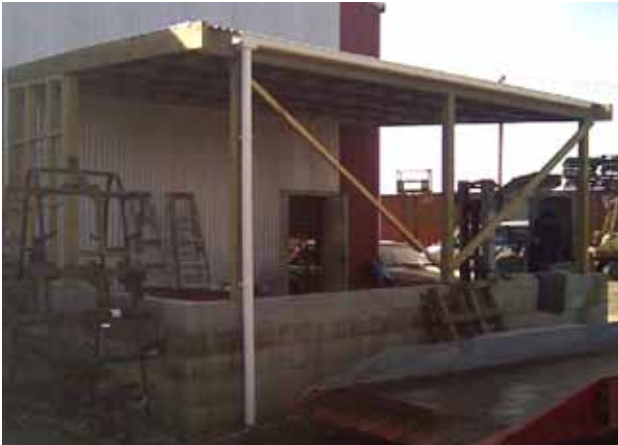
(Above) a simple roof covers a bunded wash down area
