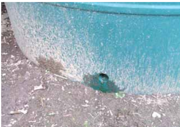
(Above) a hole drilled into a bund wall to drain rainwater making the bund completely ineffective.
