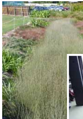
(Above and below) wetlands, swales and rain gardens can be effective and low cost options for treating stormwater run-off. These can be retrofitted to industrial sites in many cases.
