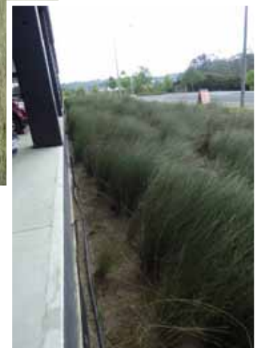
(Above and below) wetlands, swales and rain gardens can be effective and low cost options for treating stormwater run-off. These can be retrofitted to industrial sites in many cases.
