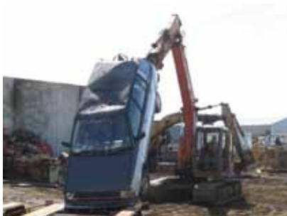
(Above) a vehicle wreck is unloaded over bare soil on a site resulting in pollution of the land.
