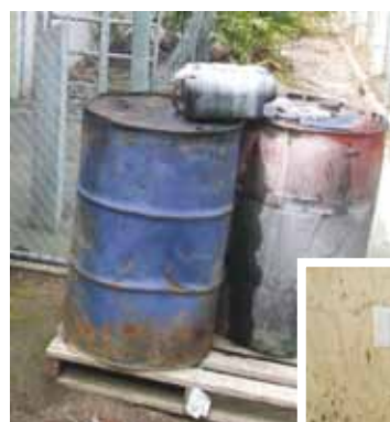
(Above) two drums used to store waste oil. This is a very poor set up due to the risk of spills and vandalism. Drums are not ideal for storage of waste oil. These should at least be bunded and under cover. A funnel should be used for filling.
