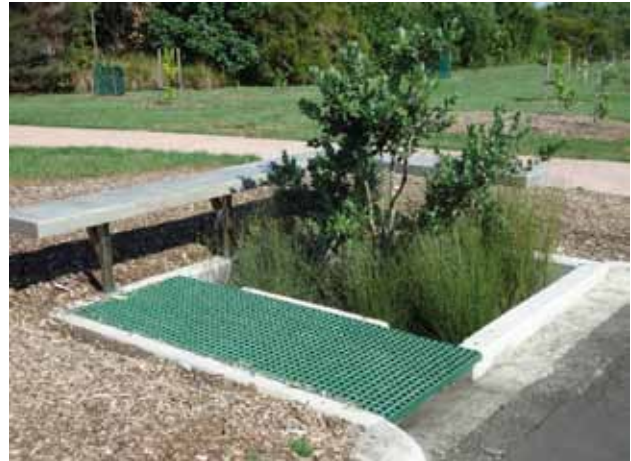
(Above) a tree pit can be used to filter stormwater run-off
