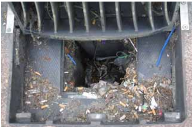
(Above) a catch pit or sump filter bag can be used to trap sediments and larger debris. The majority of filters are not suitable for run-off with high or low pH, hydrocarbons or dissolved heavy metals.
