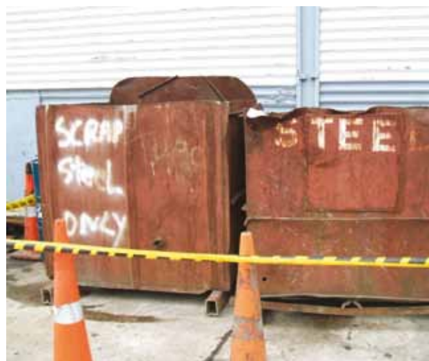
(Above) scrap steel bins are labelled correctly but should have lids to prevent rain flushing contaminants away.
