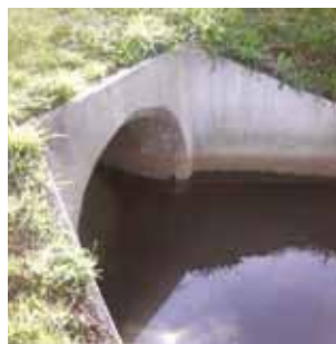
(Below) stormwater outfalls. Your staff should know where your stormwater discharges to and how to access this point in the event of a discharge or spillage.
