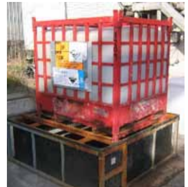
(Above) IBC on a portable bund which is good practice and would contain a leak
