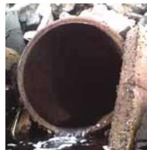
(Below) stormwater outfalls. Your staff should know where your stormwater discharges to and how to access this point in the event of a discharge or spillage.
