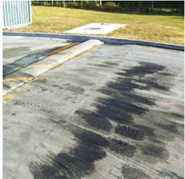
(Above) spills to a refuelling pad cause tracking of contaminants resulting in polluted stormwater runoff. Refuelling hoses should be checked regularly and spills cleaned up as they occur.
