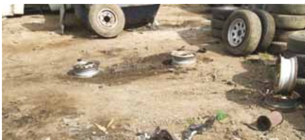
(Above) bare soil on sites will result in sediment (and other contaminants) being washed into stormwater drains. Bare soil should be sealed (with appropriate stormwater disposal installed).
