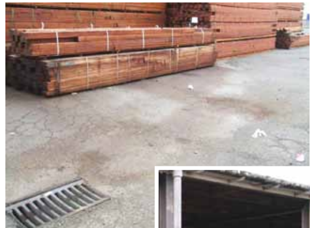
(Above) a newly treated timber stockpile leaches contaminants which are washed into a stormwater drain by rain. Treated timber should be covered or stored indoors.
