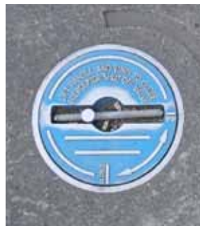
(Above and below) interceptors and shut-off valves, including signage.
