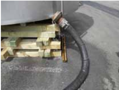
(Above) a pump hose for loading of product leaks onto hard stand leading to stormwater. Loading areas like this should be isolated to contain spills.
