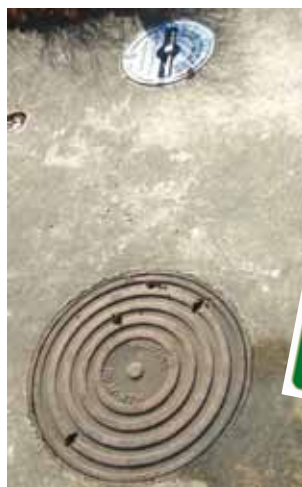
(Below) stormwater outfalls. Your staff should know where your stormwater discharges to and how to access this point in the event of a discharge or spillage.
