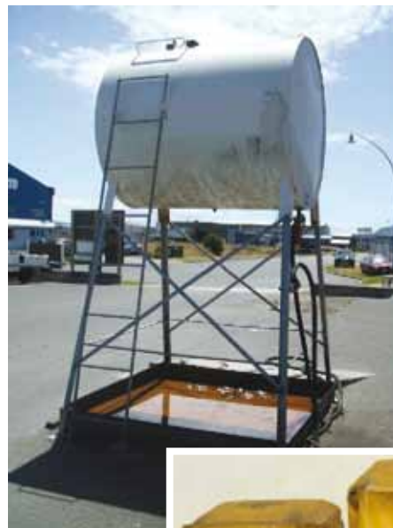
(Above) spills to a refuelling pad cause tracking of contaminants resulting in polluted stormwater runoff. Refuelling hoses should be checked regularly and spills cleaned up as they occur.
