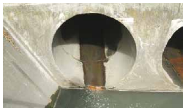
(Above and top) a process wastewater overflow pipe discharges wastewater to a stormwater grate (this is shown on the plan as connected to sewer but is in fact connected to stormwater). Wastewater discharges to an open drain leading to the harbour. Always check connections – never assume a drainage plan is correct unless it has been checked by a drain layer.
