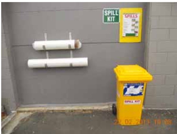
(Above) a spill station set up with kit and appropriate signage
