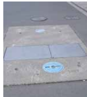
(Above and below) interceptors and shut-off valves, including signage.
