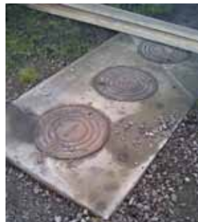
(Above and below) interceptors and shut-off valves, including signage.
