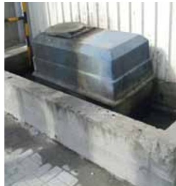
(Above) waste oil tank is well bunded but should be roofed to prevent rainwater filling the bund
