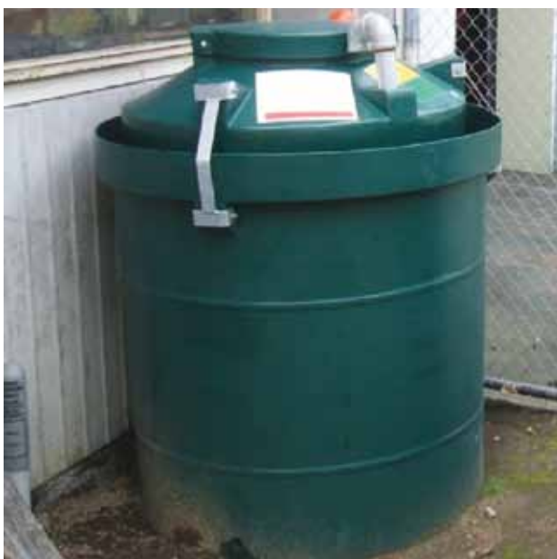
(Above) a waste oil igloo is a perfect storage solution for waste oil. This one should ideally be sited on a paved surface and under a roof.
