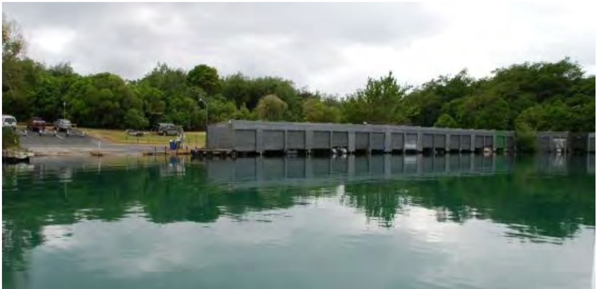
Figure 31: Strip of approximately 25 commercial style boat houses at Boatshed Bay, Lake Tarawera.
