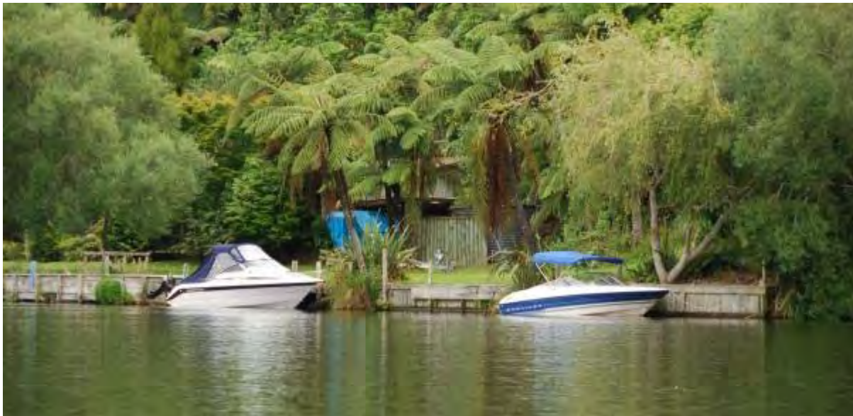
Figure 21: Okere Arm, Lake Rotoiti: Lakeshore wall doubles as marina wharf in an excavated embayment.
