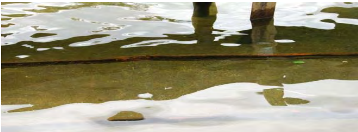
Figure 44: Typical slipway rail, partly hidden under water.
