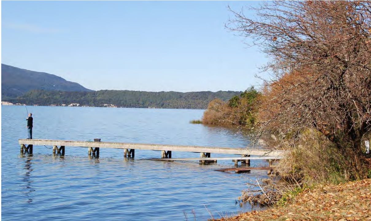
Figure 32: Jetty with adjoining slipway and rails at Lake Tarawera.
