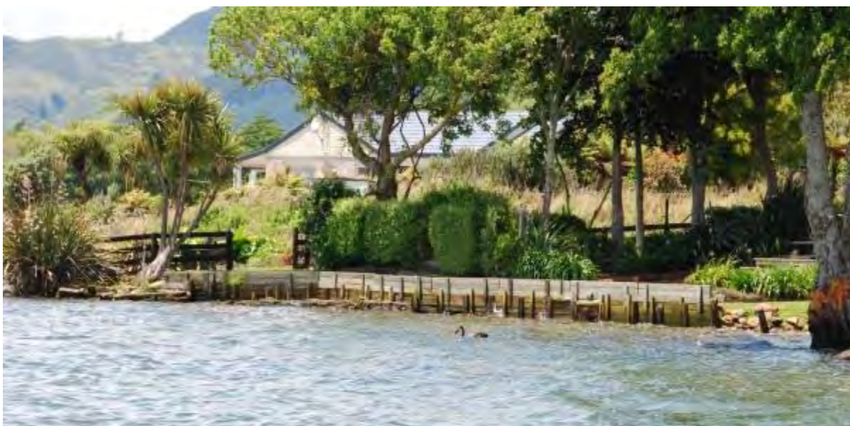
Figure 22: Hinemoa Point, Lake Rotorua: shoreline wall of rock rip rap and timber to protect against wave action.
