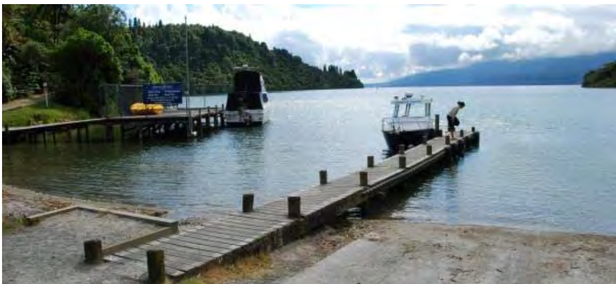
Figure 33: Private commercial jetty and board walk at left, with public boat ramp and jetty on right. A private commercial slipway with trolley is located between the two jetties. Te Wairoa, Lake Tarawera.
