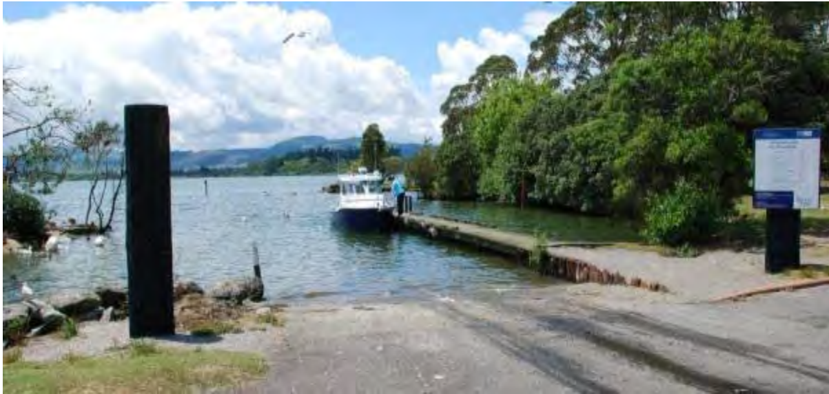
Figure 34: Public jetty and boat ramp at Sulphur Point, Lake Rotorua.
