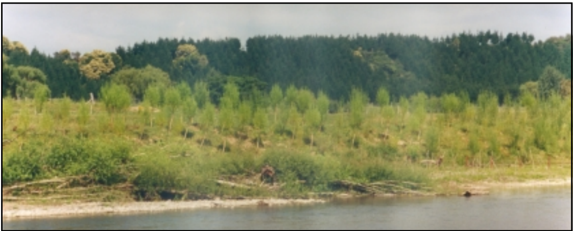
Figure 13 After - repairs utilising groyne interplanted with willow poles
