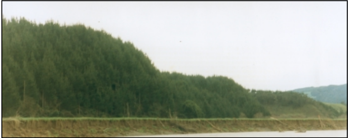
Figure 12 Before - note flood damage/severe bank erosion
