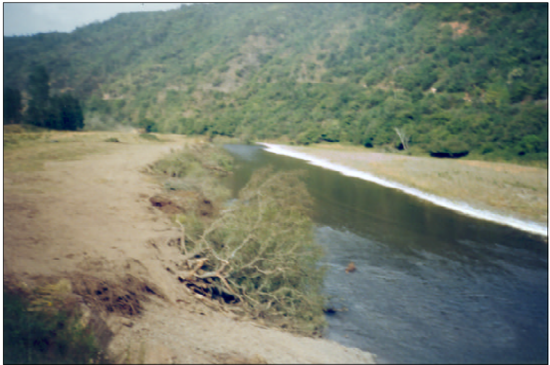
Figure 2 Willows trenched and tied to anchors - 1997 (Same site as Figure 1)
