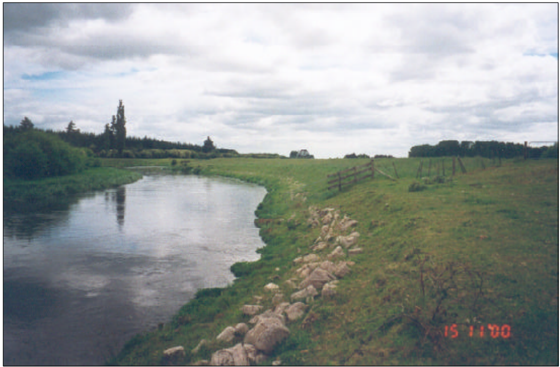
Figure 16 Rock riprap after a few years vegetation growth
