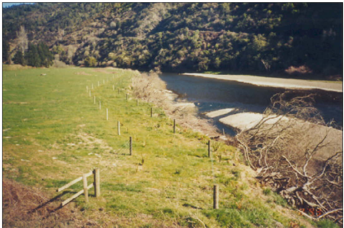
Figure 3 Buffer zone fencing to protect native shrubs - 1997 (Same site as Figure 1)
