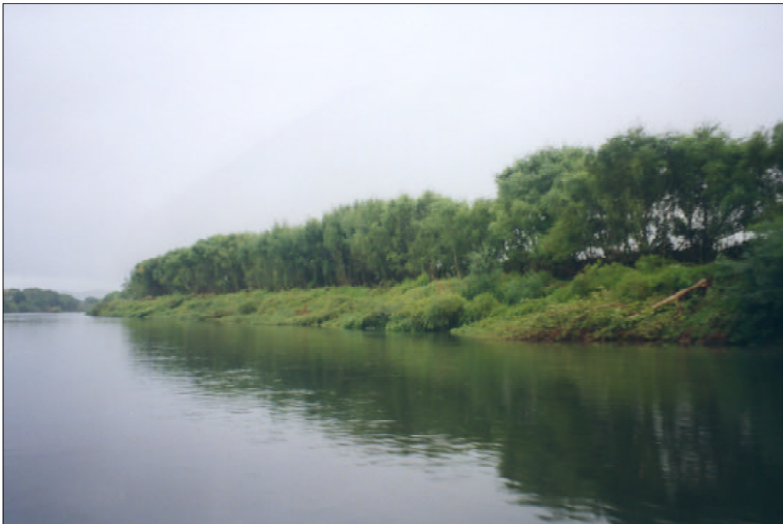
Figure 10 Willow layering - to gain a continuous vegetative edge protection
