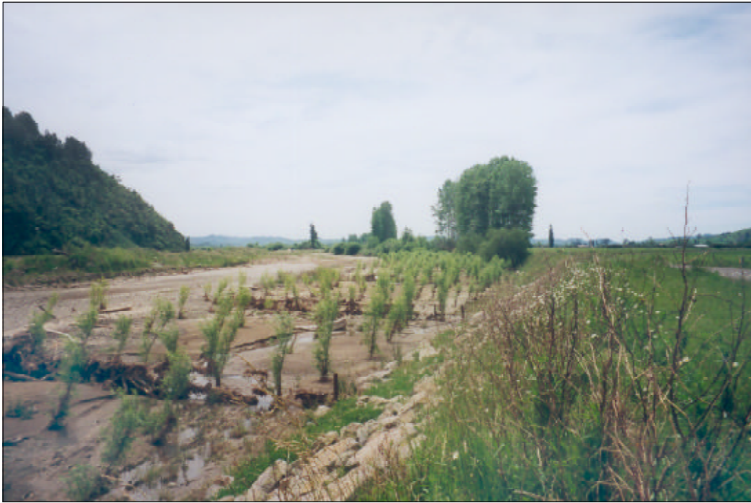
Figure 14 Aggradation of silts between training groynes with willow pole plantings and edge protection rock works. This area will become a continuous vegetative edge protection.
