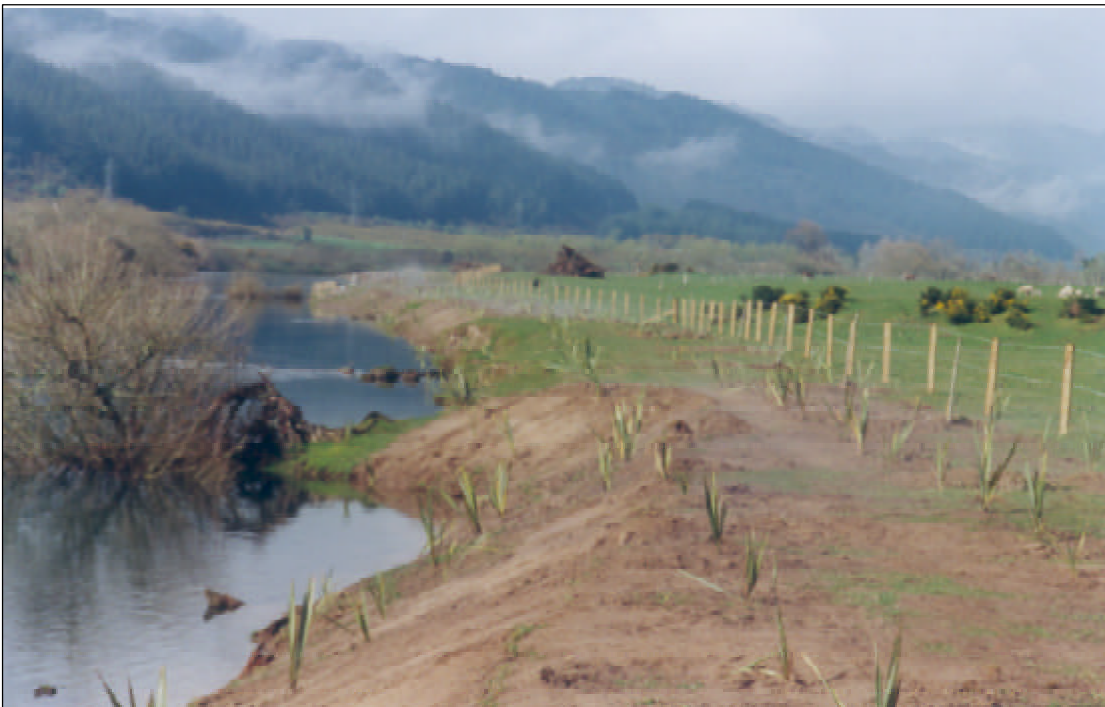
Figure 5 Battered bank with buffer zone/edge protection planting native flax
