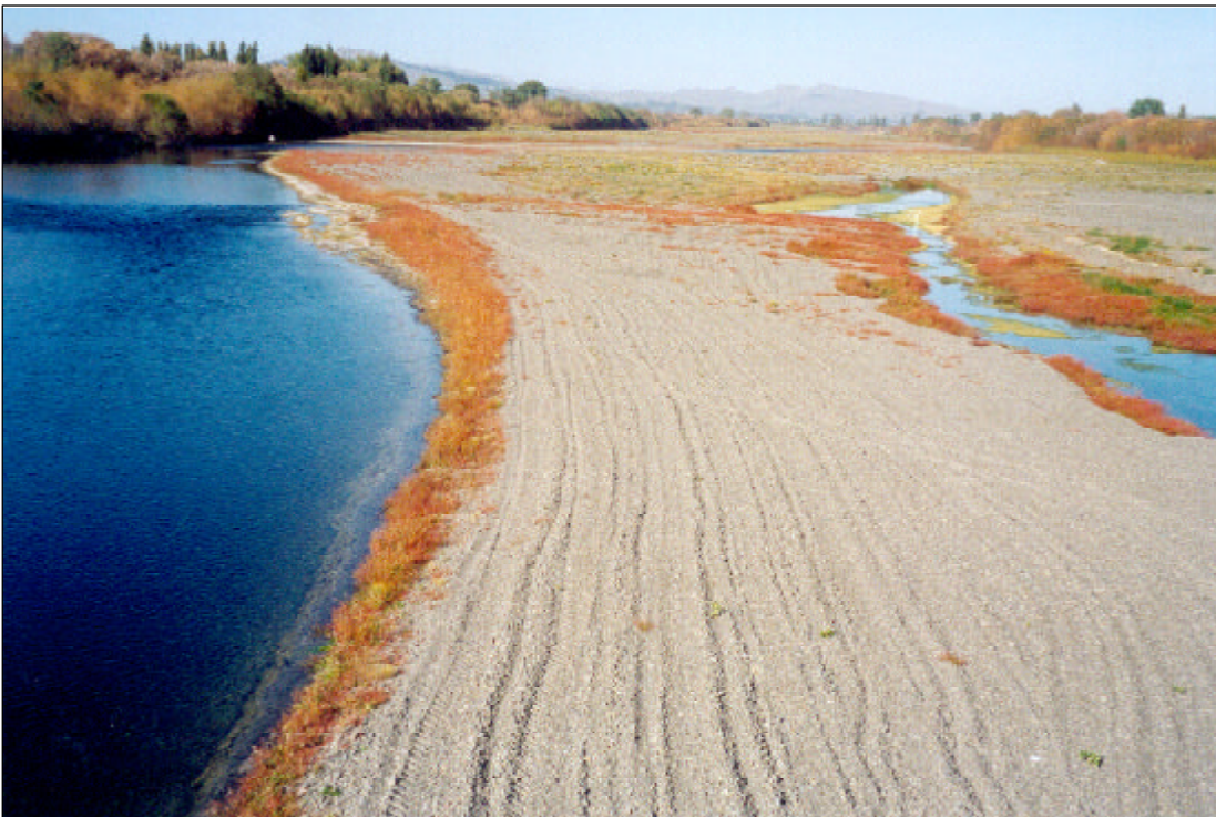
Figure 18 Beach blading/ripping
