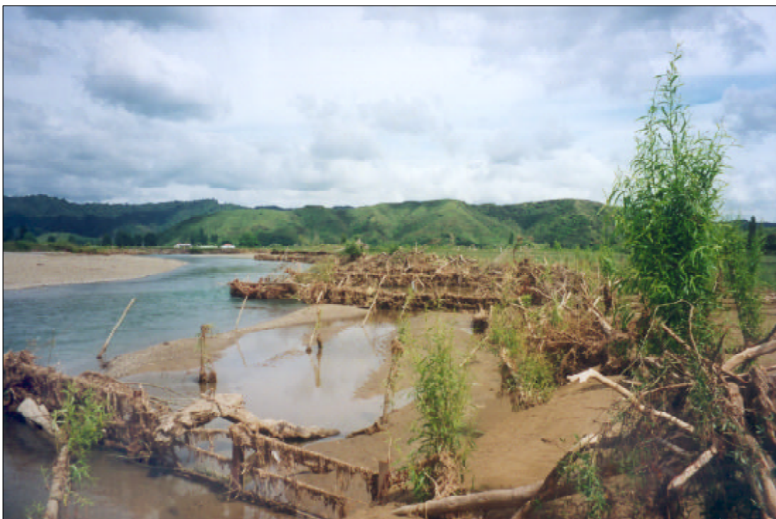
Figure 15 River training groynes - rail iron and wire rope fences constructed to stop debris and silts
