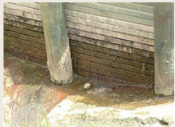
Weeping wall system showing solids retained by the wall and liquid seeping into pond.
