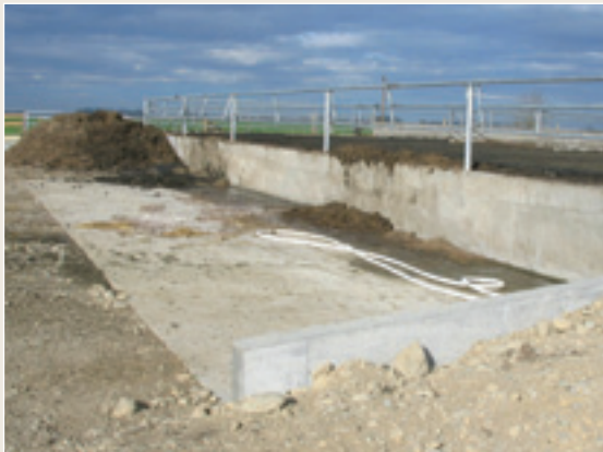
Scrapings from feed pads must be stored on a sealed, bunded area.
