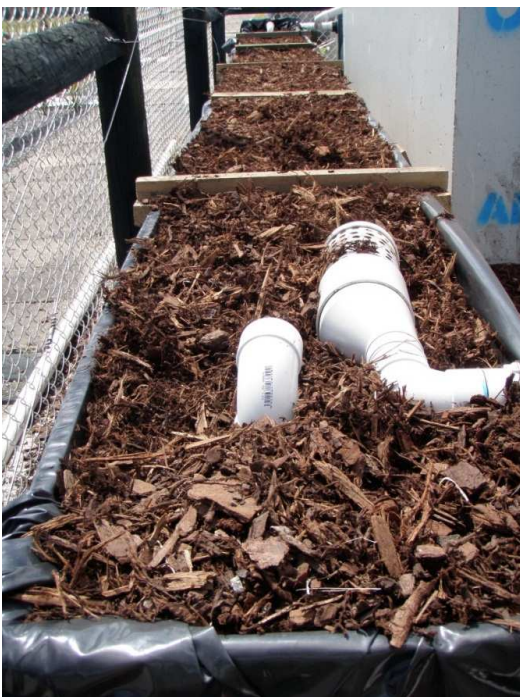
Figure 5: Bark Flume for Denitrification
