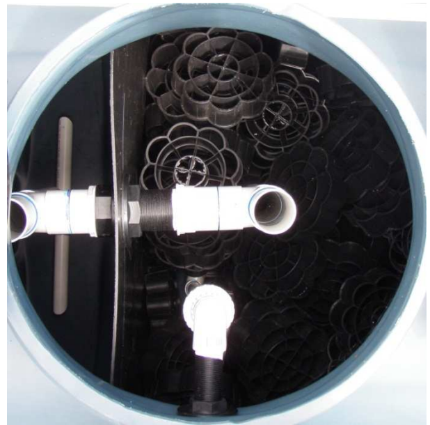
Figure 4: AWTS- N1 Inside view of treatment tank
