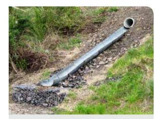
Flume drop structure with energy dissipater as an outlet control
