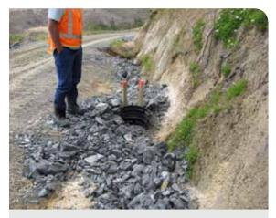
Check dam – formed from plastic fluming and graded rock
