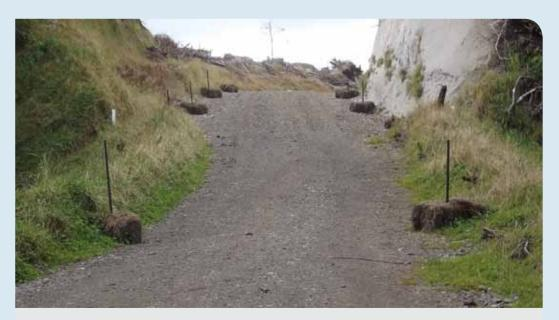
This forestry road has a range of controls in the water tables, including metalling, grassing and using hay bales to slow down the speed of the water flow.
