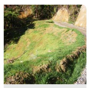
Surface stabilisation of this batter slope has been achieved by hydroseeding
