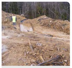
Sediment trap has been installed in stable ground. Discharge is through a flume over the batter slope
