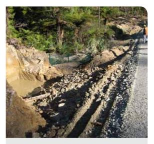
Soak hole plus silt fence where the discharge point is close to a stream
