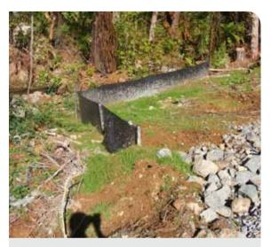
Silt fence used to intercept diffuse runoff from road, and trap sediment on site
