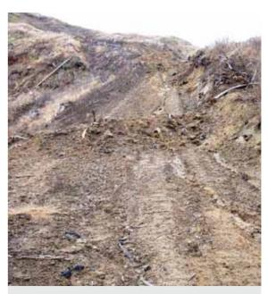
Cut off installed on haul track diverting water onto stable outfall area.
