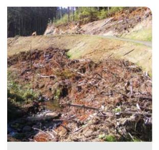
Combination of hydroseeding, grassing and slash to stabilise ground surface and help filter any sediment before reaching stream channel
